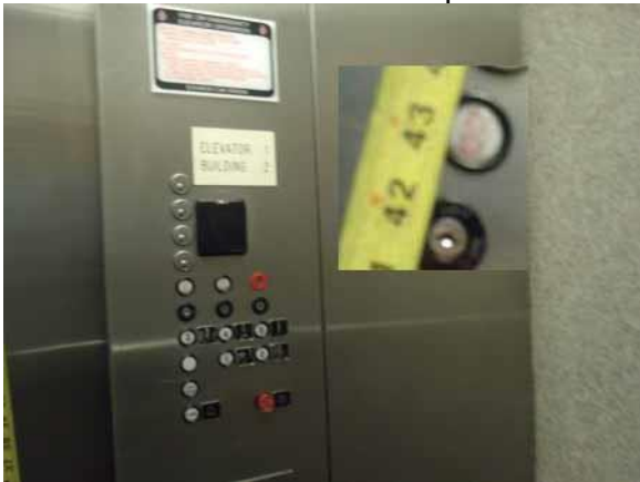
This control height is compliant
