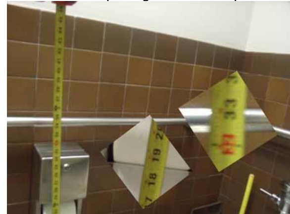
These heights are compliant
