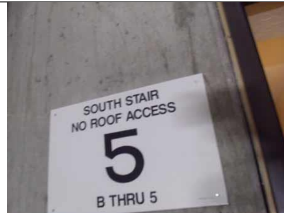
Provide proper floor identification signage
