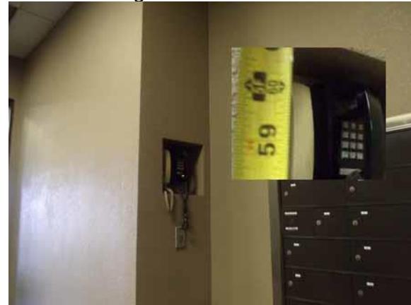
The 2 way communication phone exceeds 48" high
