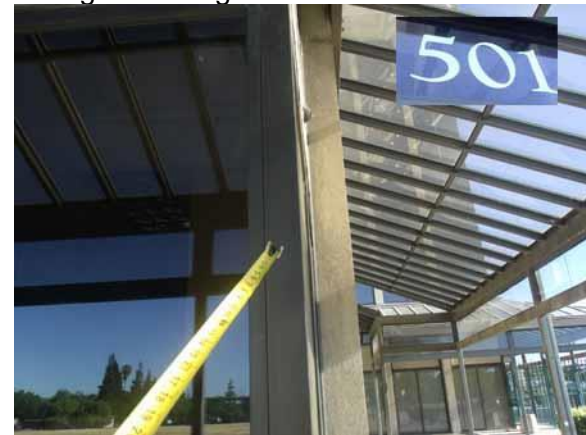
Provide sign directing to the accessible route/entrance
