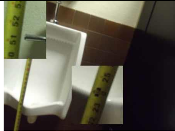
Urinals shall be 17" maximum high to top of the rim
