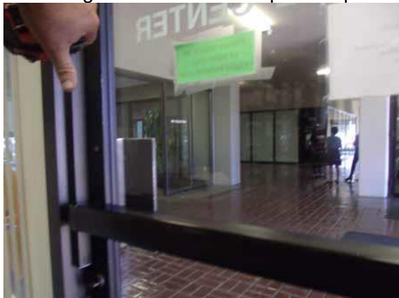
This door operation forces exceed allowable
