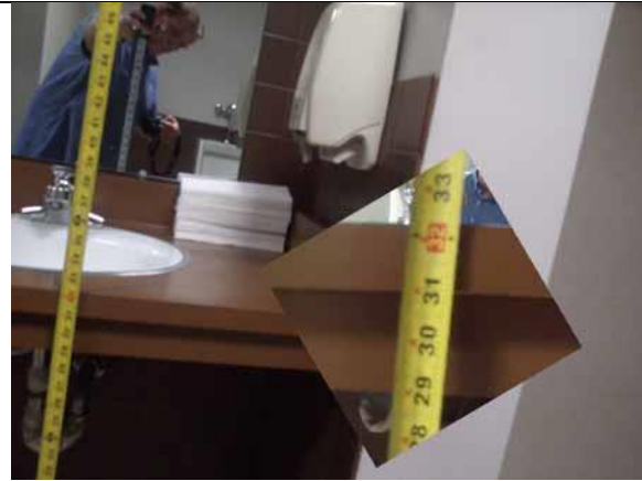
Provide proper knee clearance under the lav
