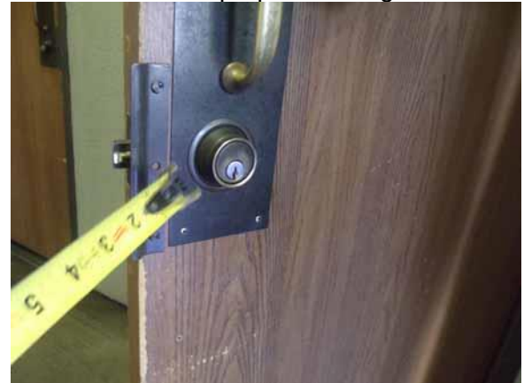
This key lock requires pinching and twisting to operate
