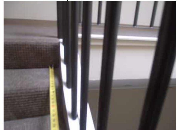
Properly stripe the edge of the top and bottom risers
