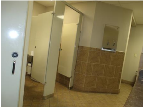
Overall exit shot
