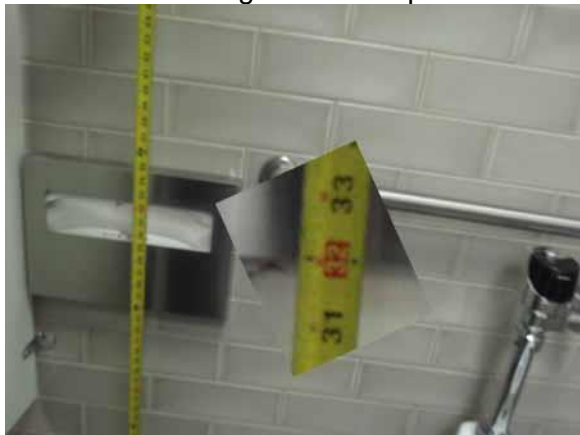
This toilet seat cover height is compliant
