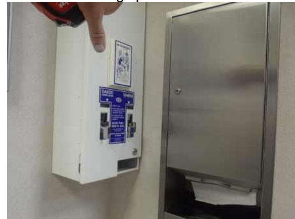
These controls require pinching and twisting to operate
