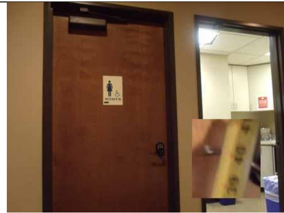
This door handle height is compliant
