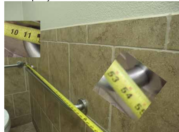
This side grab bar location is compliant
