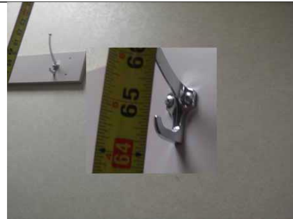
Provide a coat hook at 48" maximum high
