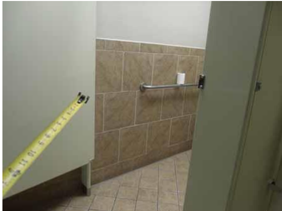
Stall door shall be self-closing
