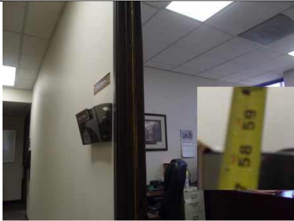
Provide cane detection or replace with thinner basket
