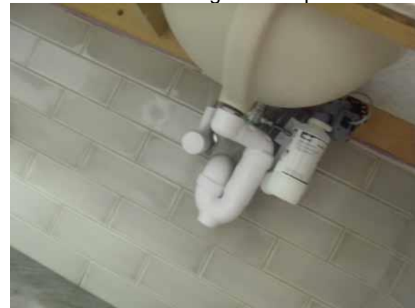
This plumbing protection is compliant
