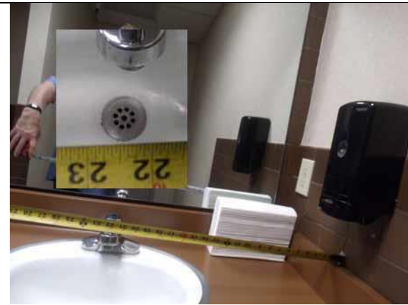
This lav offset is compliant
