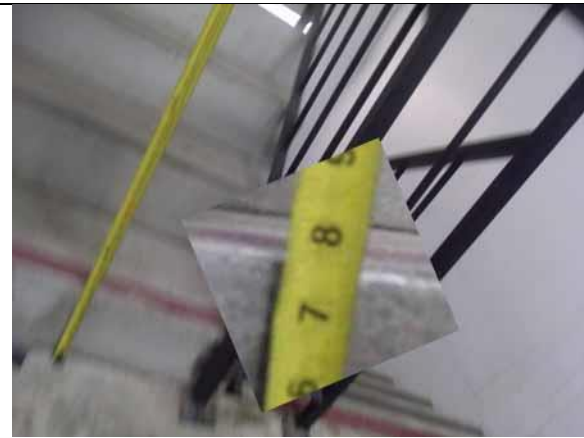
This riser height is compliant
