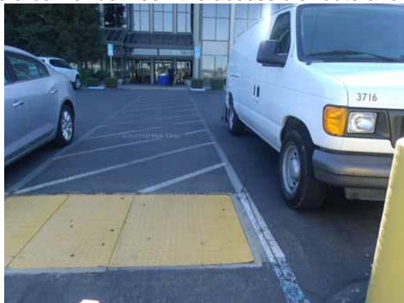
Remove the domes in the vehicular area
