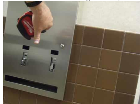
These controls require twisting and pinching to operate
