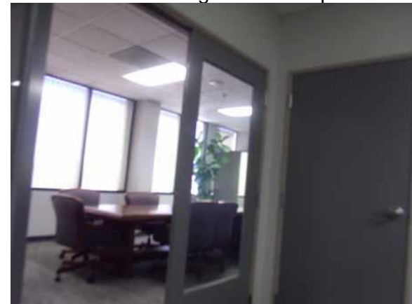
Maintain clear opening widths of 32" minimum clear
