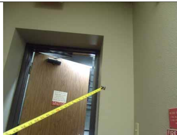
Provide proper stair exit braille sign
