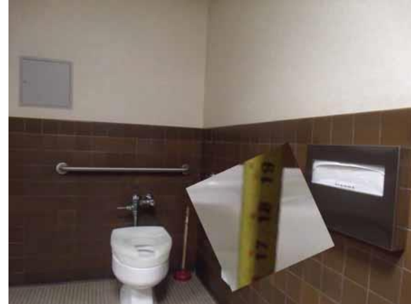
This toilet seat height is compliant
