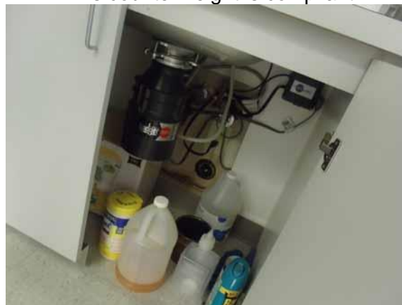
Knee clearance is not required without a cook top appliance
