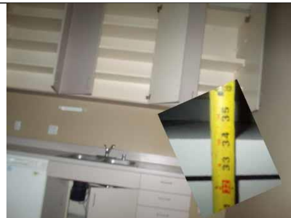
This counter height is compliant
