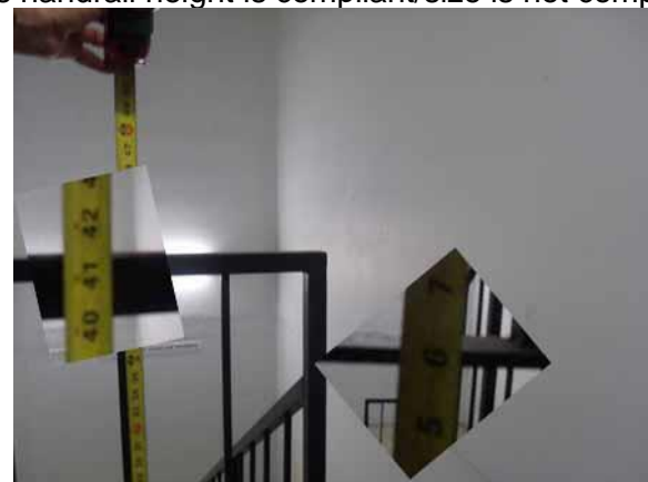
Gaurdrails is not 42" high minimum
