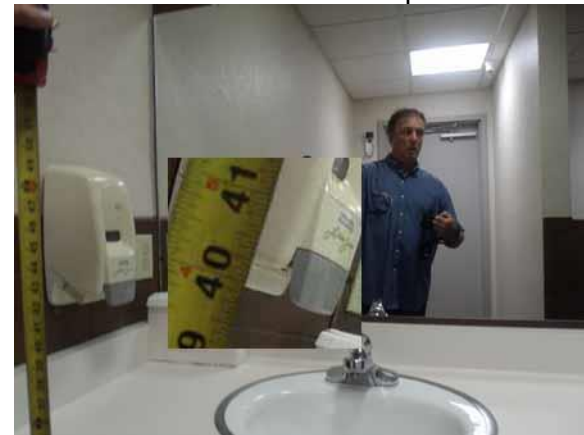
This mirror height is compliant
