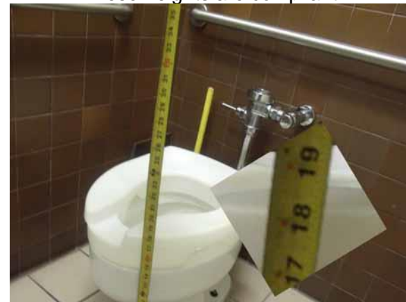
This toilet seat height is compliant
