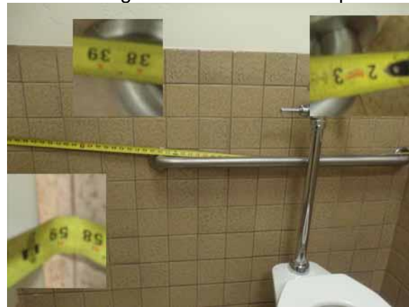
Stall width and rear grab bar location are not compliant
