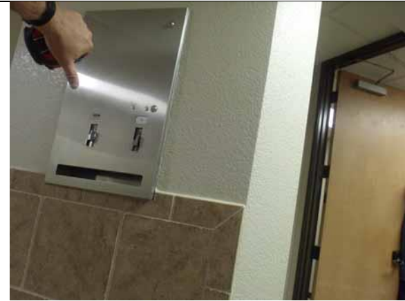
This machine requires twisting and pinching to operate
