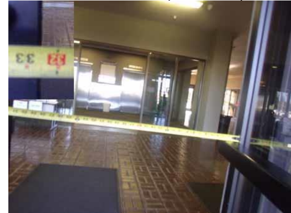
Maintain 32" minimum wide clear opening width
