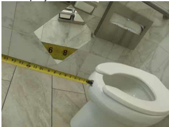
This toilet paper location is compliant
