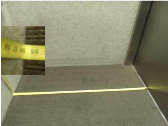
This dimension is compliant
