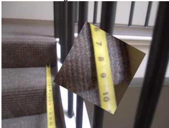
This tread depth shall be 11" minimum
