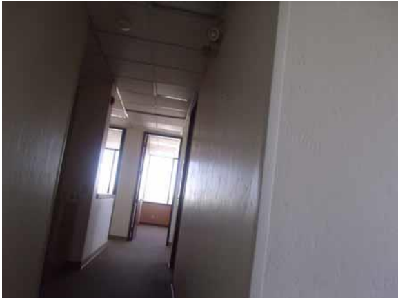
Maintain a min 44" wide route or 32" min for 24" long max
