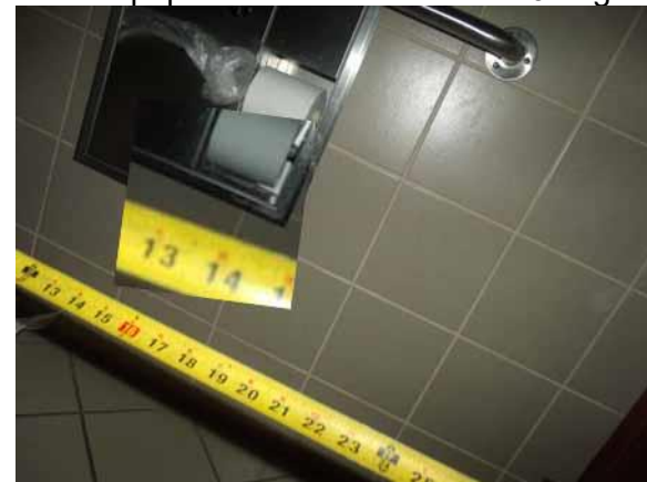
Properly locate the toilet paper dispenser
