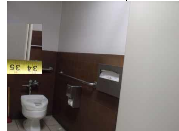
This clear opening width is compliant
