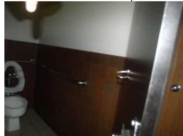
Remove stall panels and create a single user restroom
