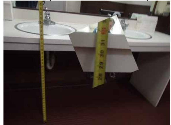
Provide proper knee clearance under the lav
