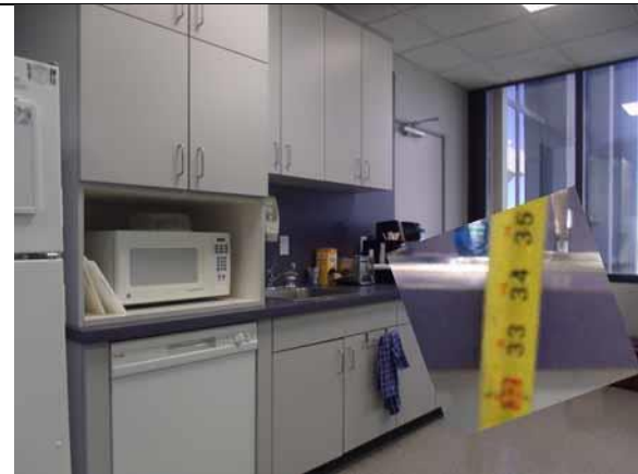
This counter height is compliant
