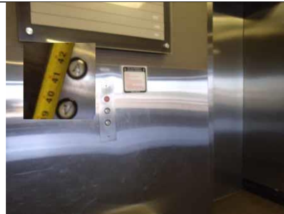
These call buttons are compliant
