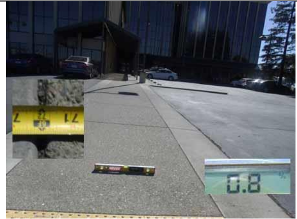
This section slope and width are compliant
