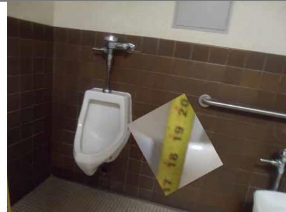
Lower the urinal to be 17" maximum high to top of rim
