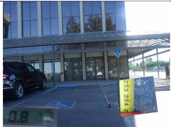
This accessible parking length and slope are compliant
