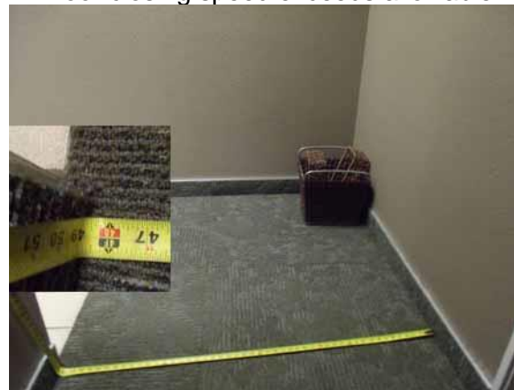
This clear floor area is compliant
