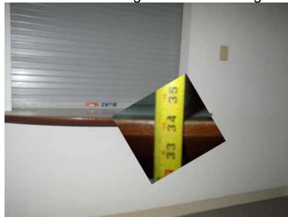
This counter height is compliant
