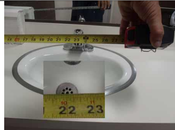
This lav offset is compliant
