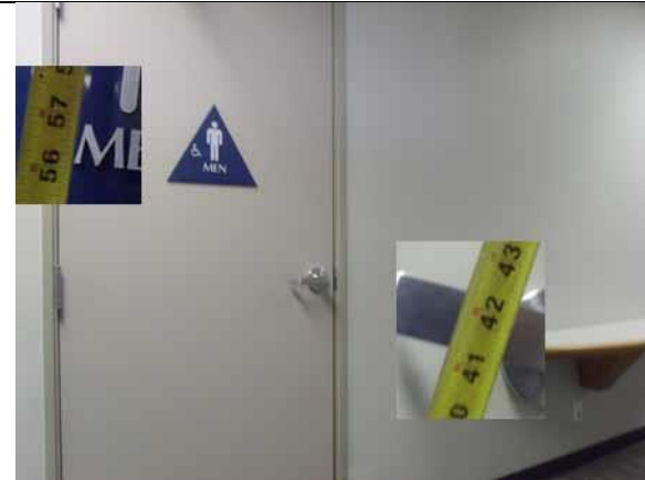
These heights are compliant
