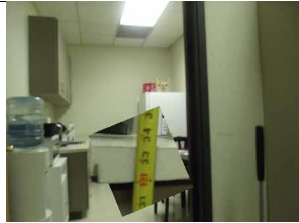
This counter height is compliant
