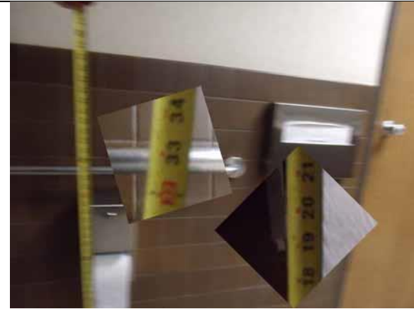
These heights are compliant
