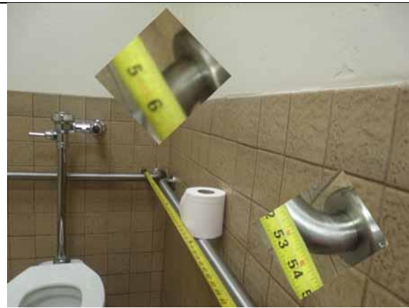
This side grab bar location is compliant
