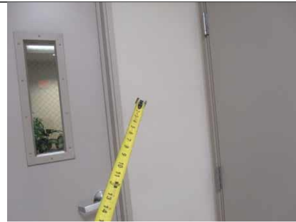
Provide proper signage for the stairs
