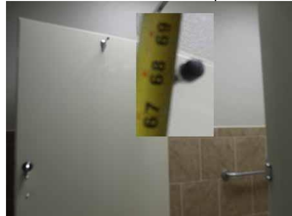
Provide a coat hook at 48" maximum high
