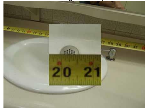
This lav offset is compliant
