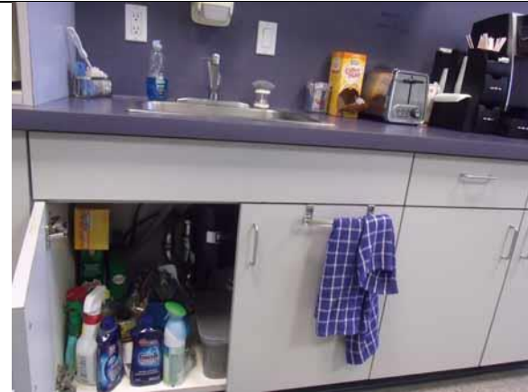
Knee and toe clearance is not required without a cooktop appliance
