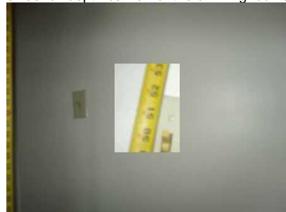
This switch height meets applicable codes
