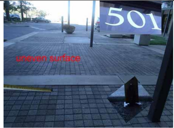
Repair the uneven surface and gap
