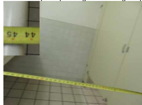
This width in front of stall door shall be 48" minimum
