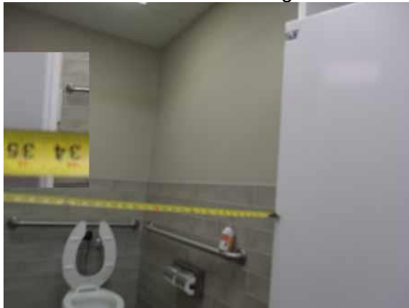
This door width is compliant
