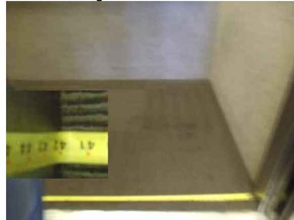
This opening width is compliant
