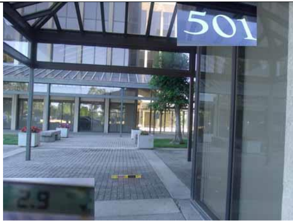
This section of cross slope exceeds 2.08%
