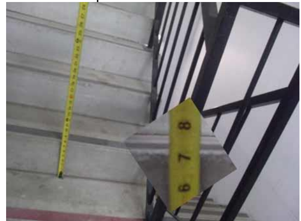
This riser height is compliant
