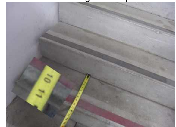
This step depth is compliant
