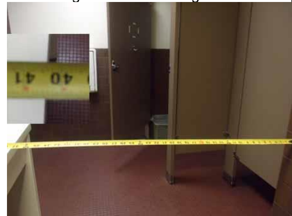
Provide a minimum 44" width to accessible stall
