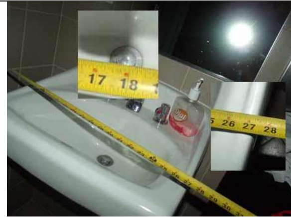
Properly offset the lav to be 18" minimum to center from wall
