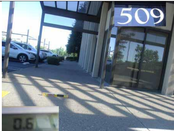
This section slope and width are compliant
