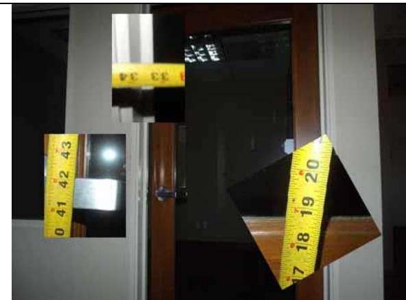
This door hardware and width are compliant
