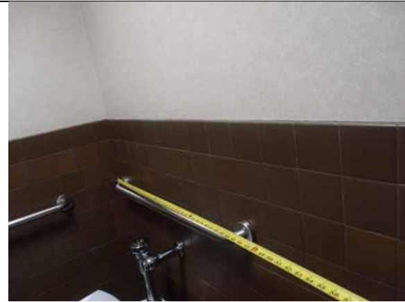
Properly locate the rear grab bar
