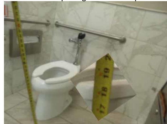
This toilet seat height is compliant
