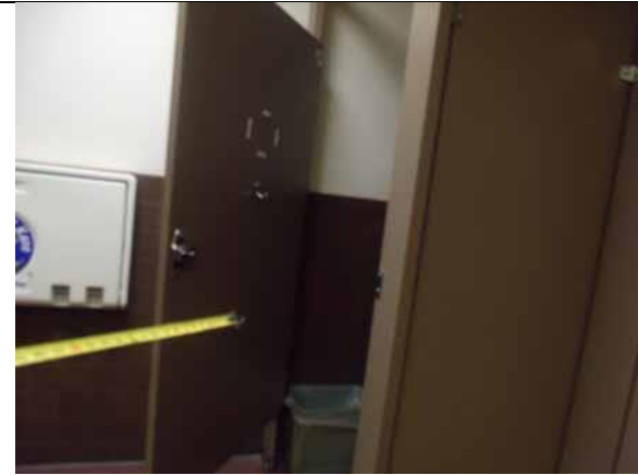
Stall door shall be self-closing typical
