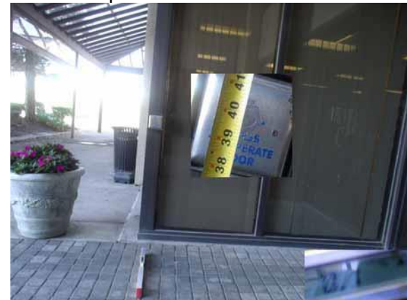
Provide a low level push pad
