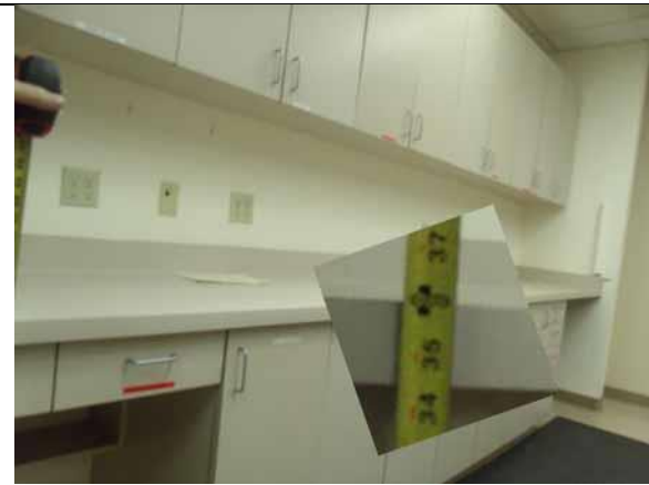
This counter height is compliant
