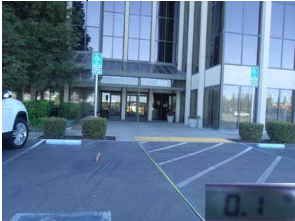
This section of slope is compliant
