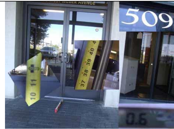
This hardware and slope are compliant
