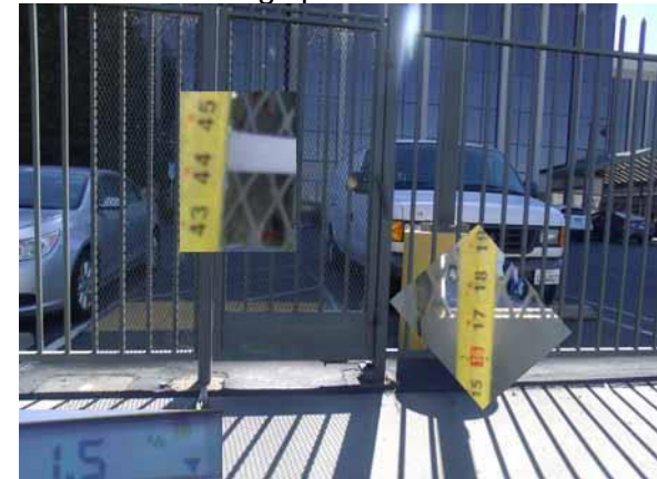
This door hardware and slope are compliant
