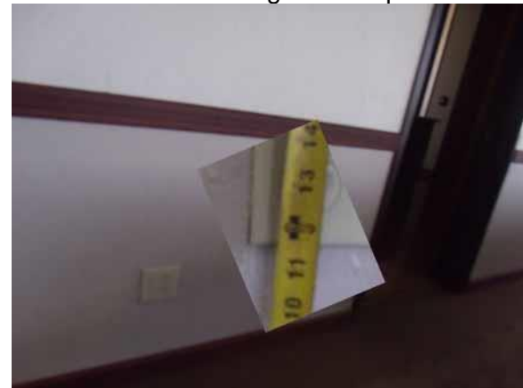
This electrical outlet height meets applicable codes
