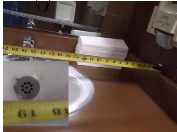
This lav offset is compliant
