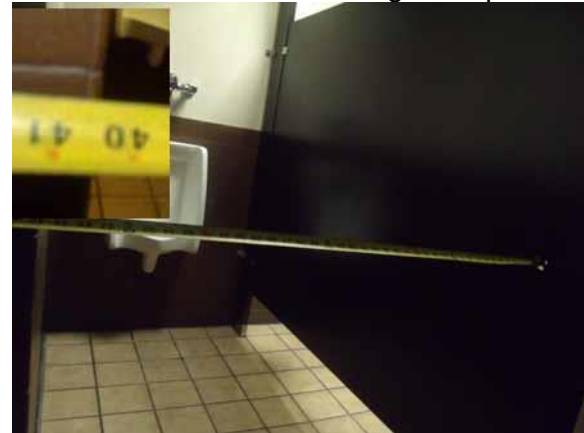
This urinal alcove width is compliant
