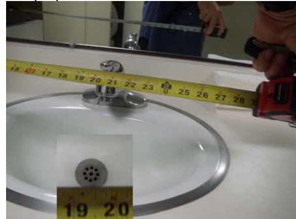
This lav offset is compliant
