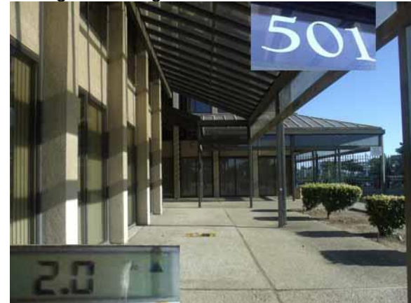
This section slope and width are compliant
