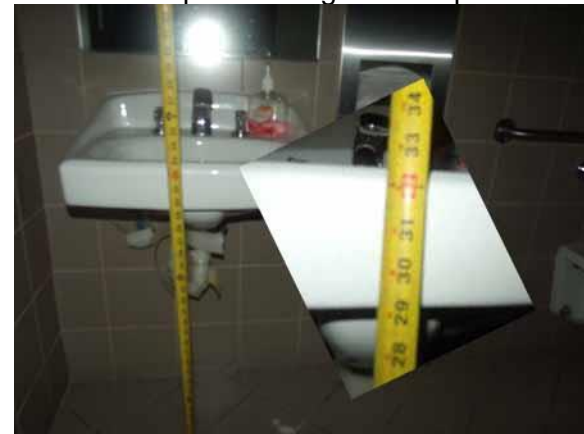
This lav height is compliant
