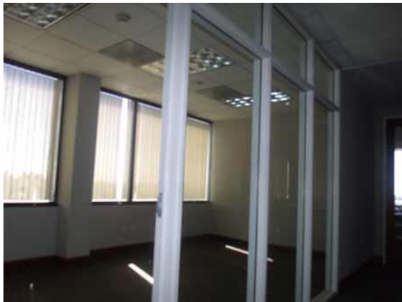
Maintain a min 36" wide route or 32" min for 24" long max
