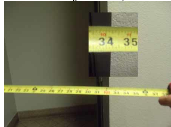
This clear opening width is compliant
