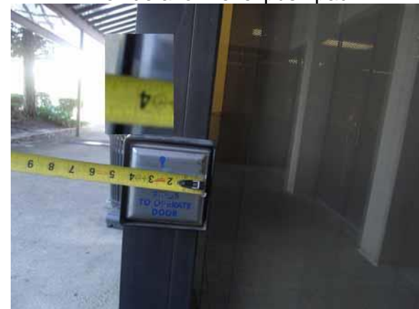
This push pad size is compliant
