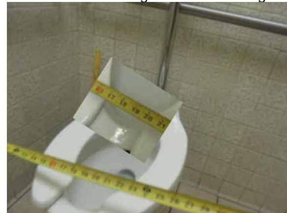
Properly offset the toilet
