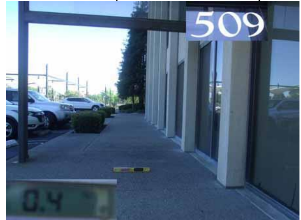
This section slope and width are compliant
