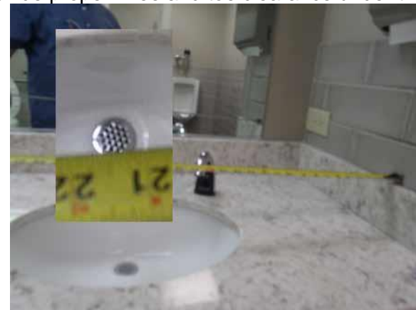
This lav offset is compliant
