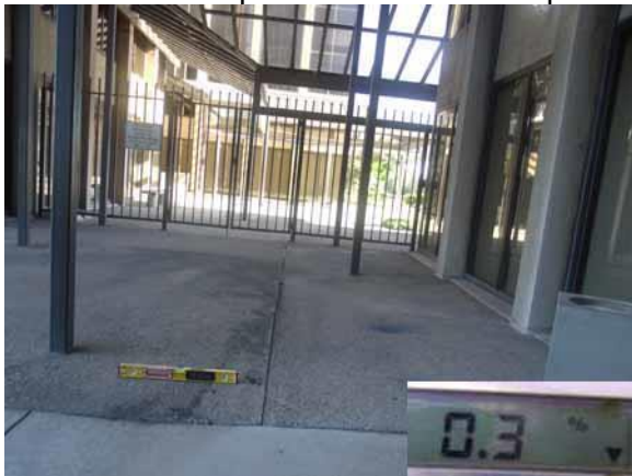
This section slope and width are compliant
