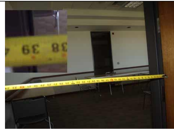
This clear opening width is compliant
