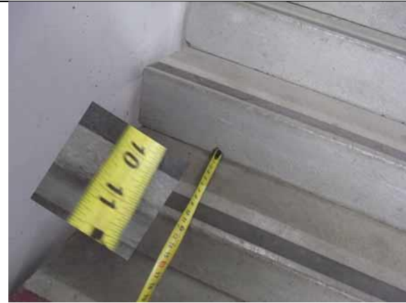
This step depth is compliant
