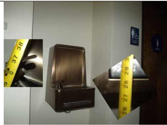
This spout height is compliant
