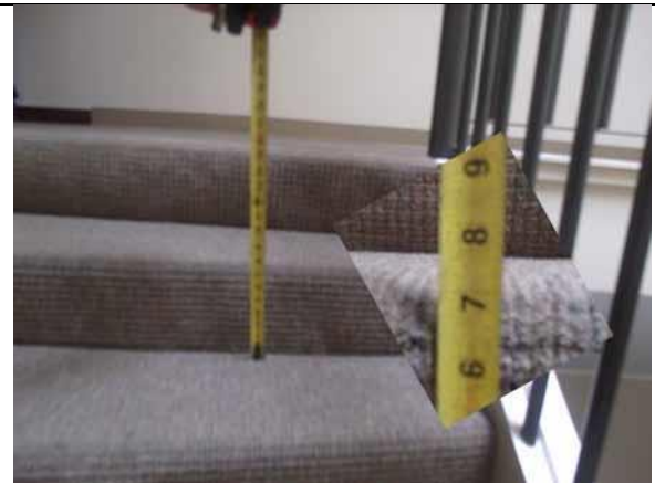
This riser height shall be 7" maximum
