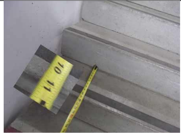
This step depth is compliant
