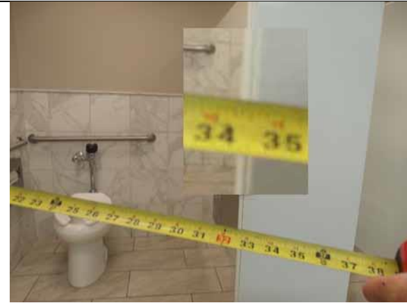
This clear opening width is compliant
