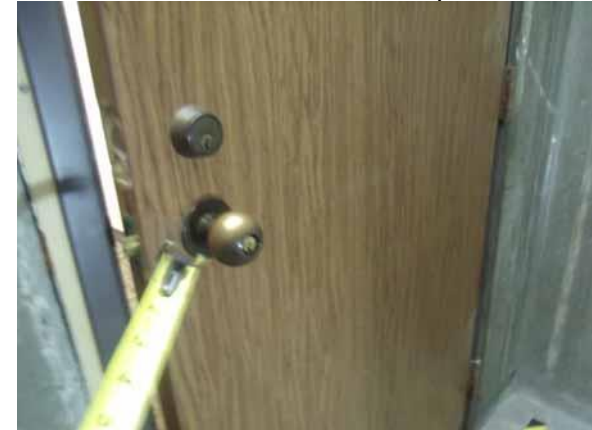
Provide lever type handles for all doors
