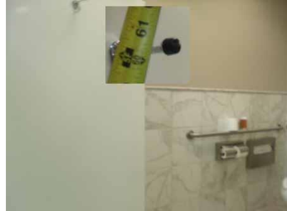
Provide a coat hook at 48" maximum high
