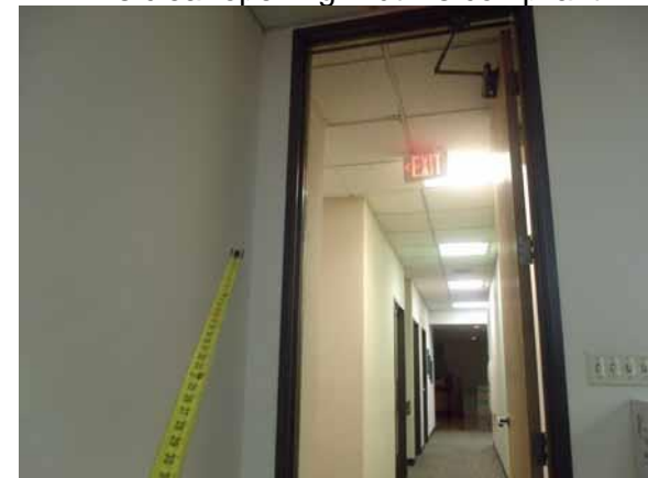
12" side clearance required with closure and latch
