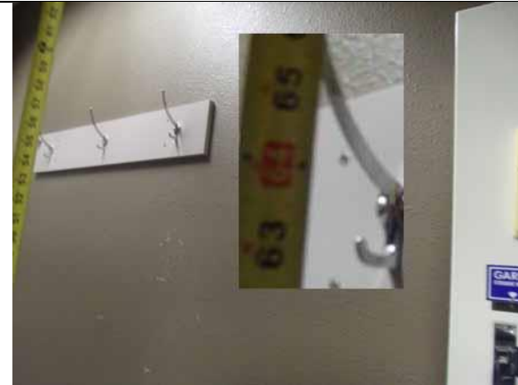
Provide a coat hook at 48" maximum high
