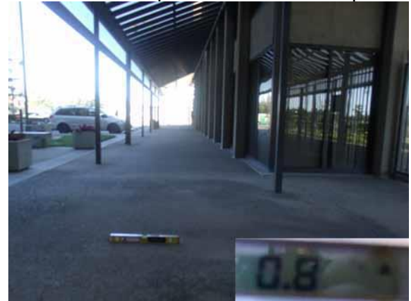
This section slope and width are compliant
