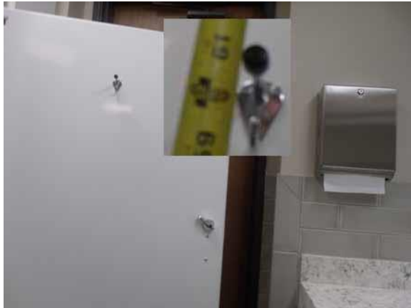
Provide a coat hook at 48" high maximum
