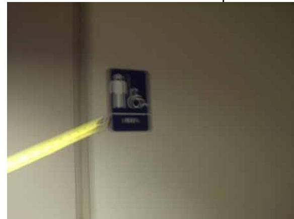
Remove the existing wall sign
