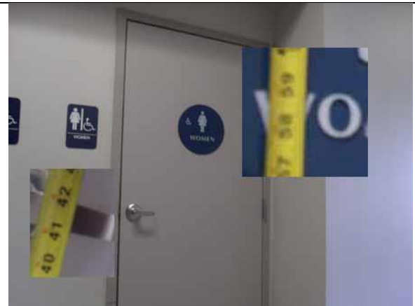
Remove the existing wall sign
