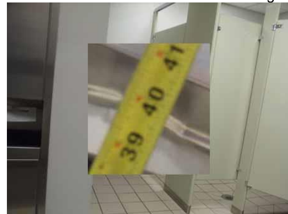
This toilet seat cover height is compliant
