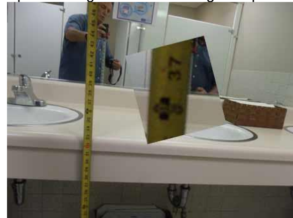
This mirror height is compliant
