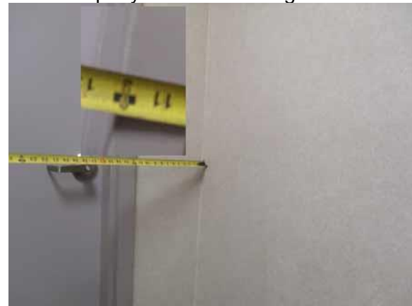
This push side clearance is compliant
