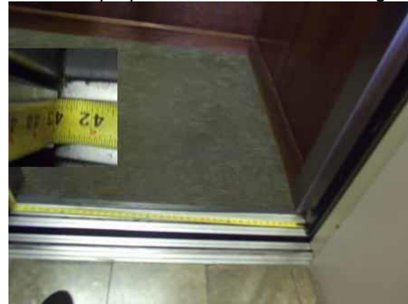
This opening width is compliant
