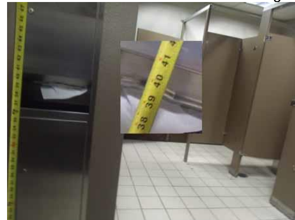
This dispenser height is compliant
