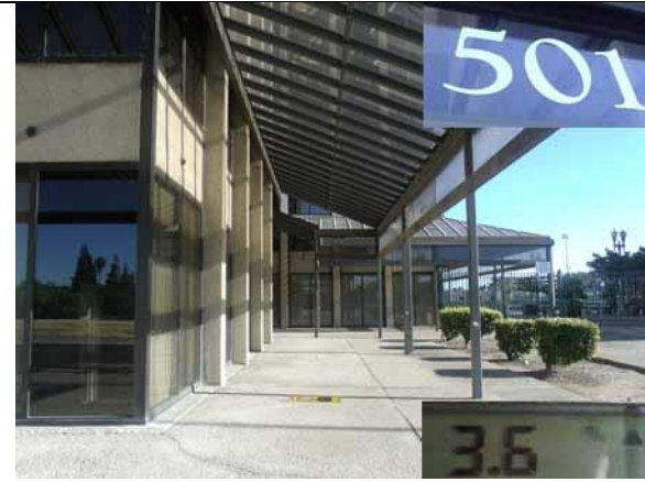
Provide sign directing to the accessible route/entrance
