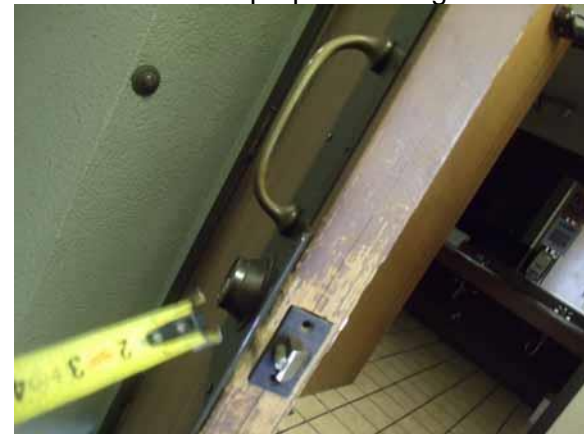
The key hardware requires pinching and twisting to operate
