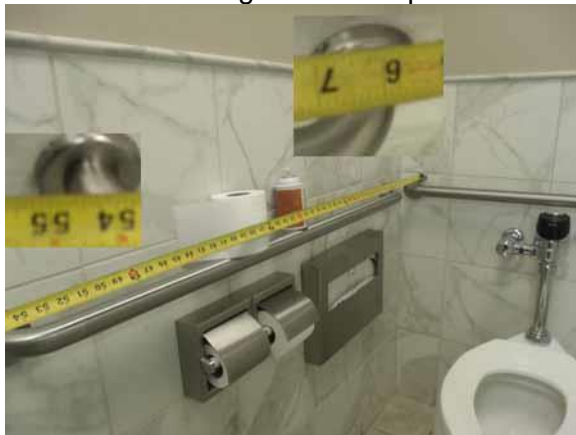
This side grab bar location is compliant
