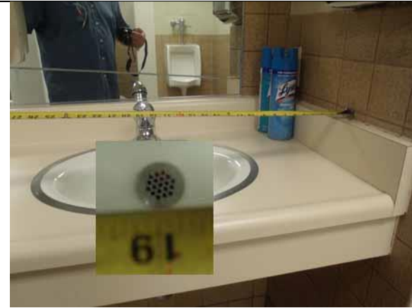
This lav offset is compliant
