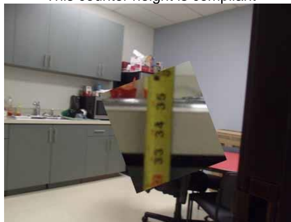
This counter height is compliant
