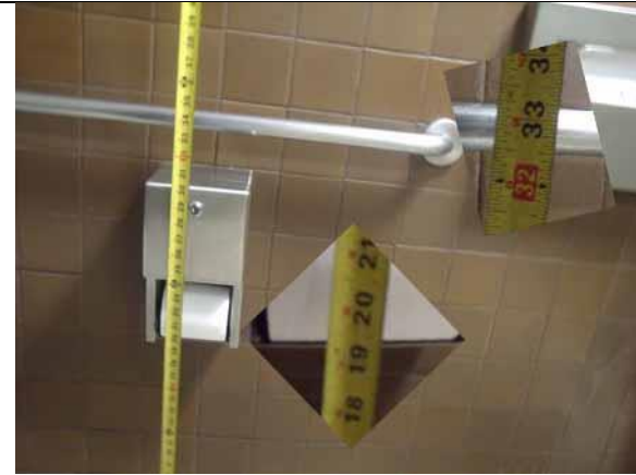
These heights are compliant
