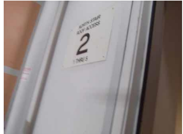
Provide proper floor Braille identification sign
