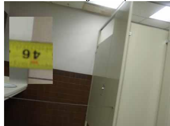
This access width is compliant
