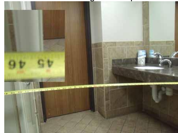
This clear width is compliant
