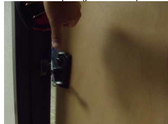
This door operation forces exceed allowable
