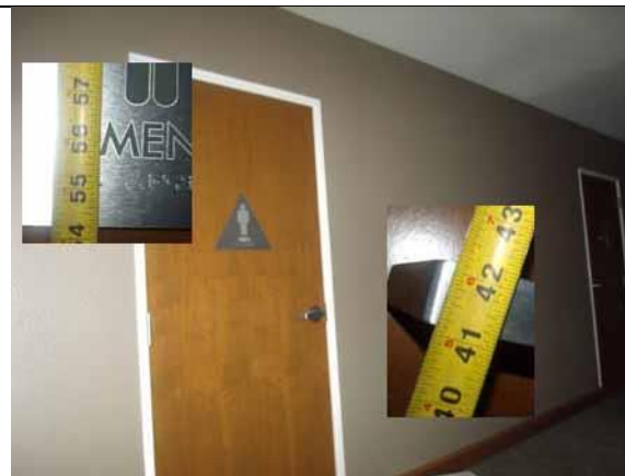
These heights are compliant
