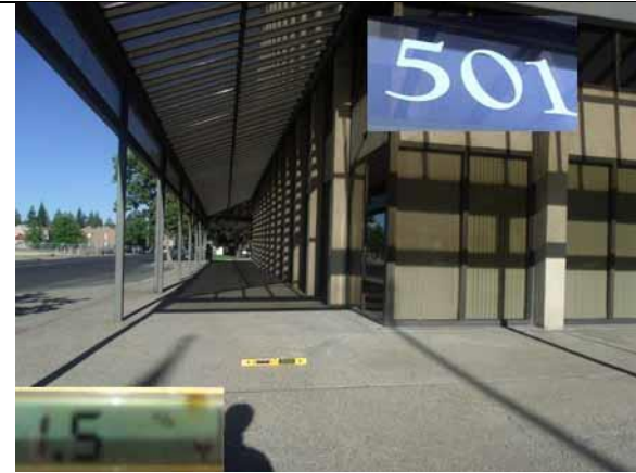
This section slope and width are compliant
