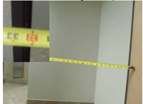
This door width is compliant
