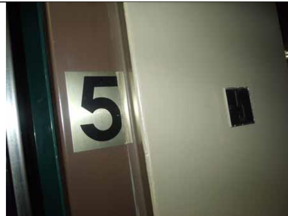
Provide proper braille number at 60" high
