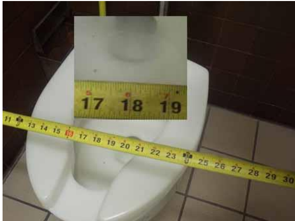
This toilet offset is compliant
