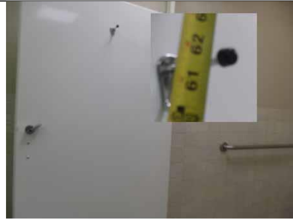
Provide a coat hook at 48" maximum high
