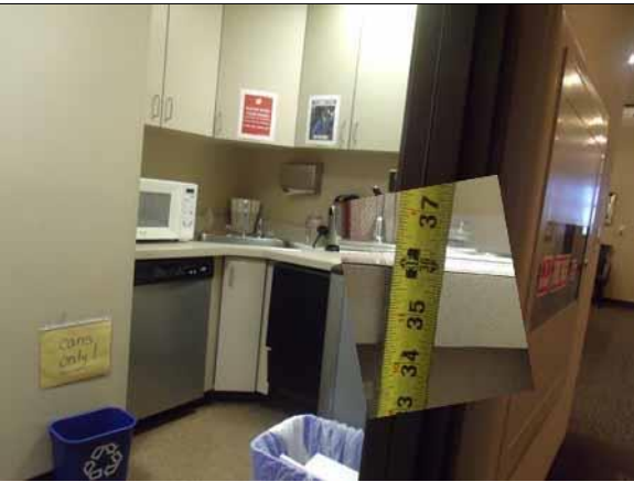
This counter height is compliant
