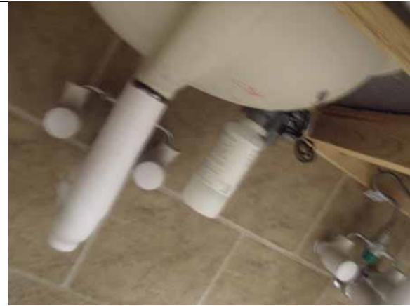
This plumbing protection is compliant
