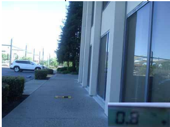
This section slope and width are compliant
