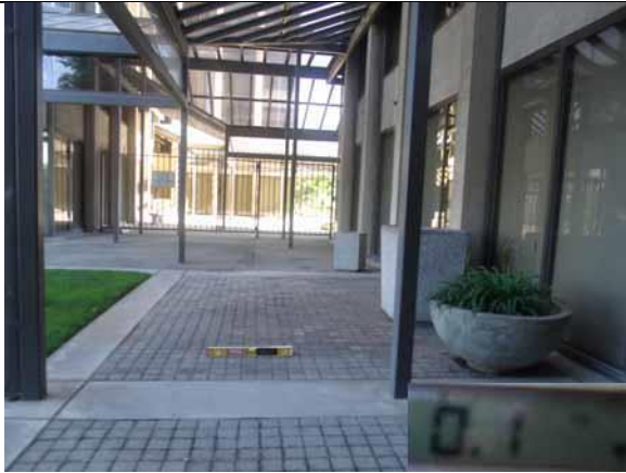
This section slope and width are compliant
