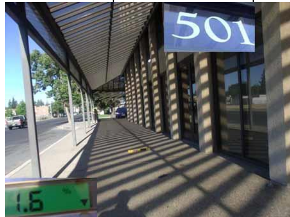
This section slope and width are compliant
