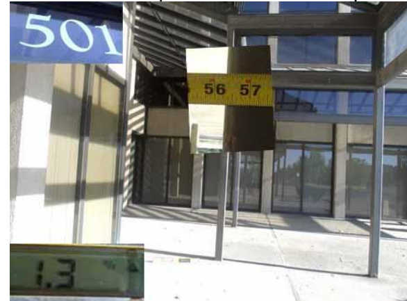
This section slope and width are compliant
