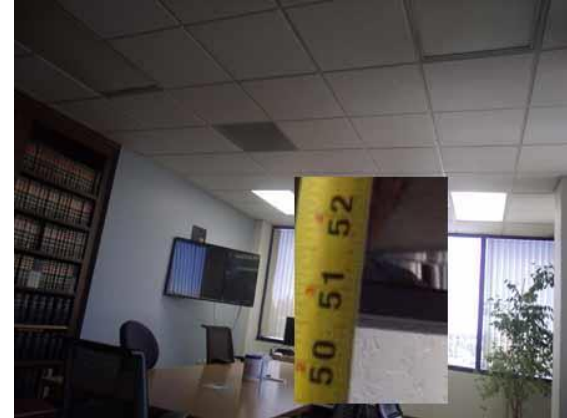
The TV is a protruding object
