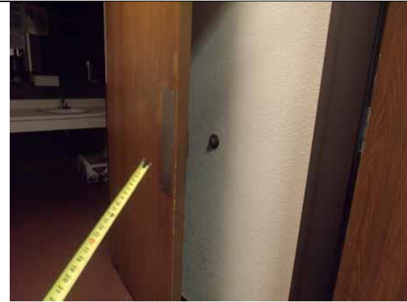
Remove the inner door swinging in series
