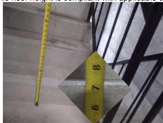
This riser height is compliant with applicable code
