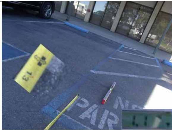
This slope and latter height are compliant
