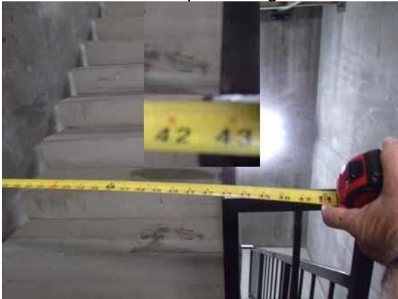
Stair width meets time of construction
