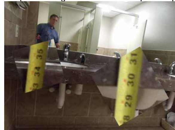
This lav height is compliant
