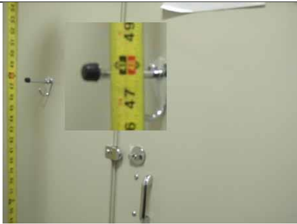
This coat hook height is compliant
