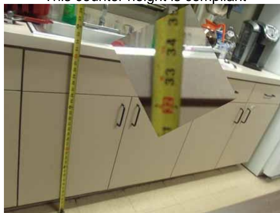
This counter height is compliant
