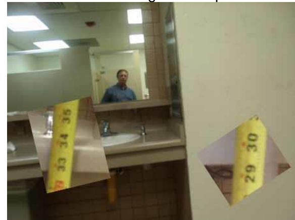
This lav height is compliant
