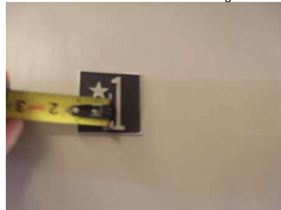
This requires a 2" star for the ground floor identification
