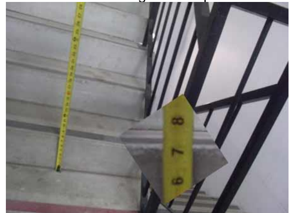
This riser height is compliant
