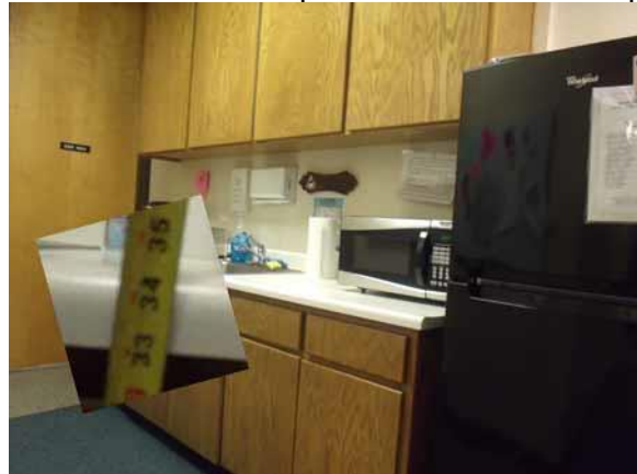
This counter height is compliant
