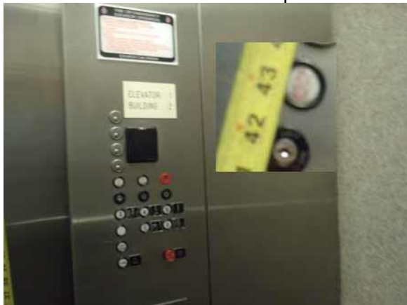
This control height is compliant
