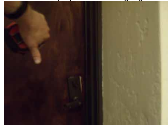
Provide proper door hardware and closing speed
