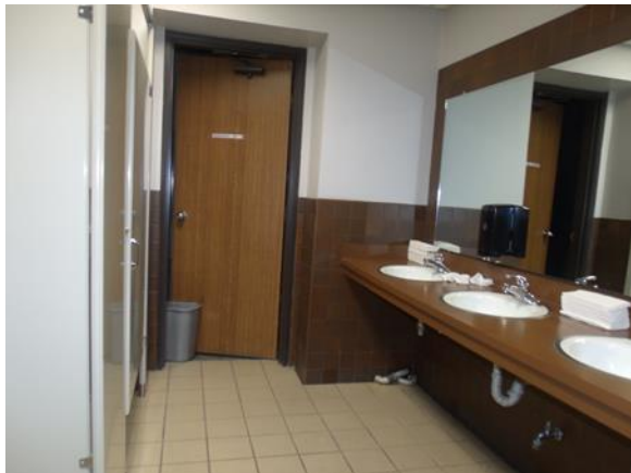
Overall Lav area
