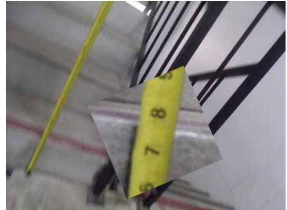
This riser height is compliant
