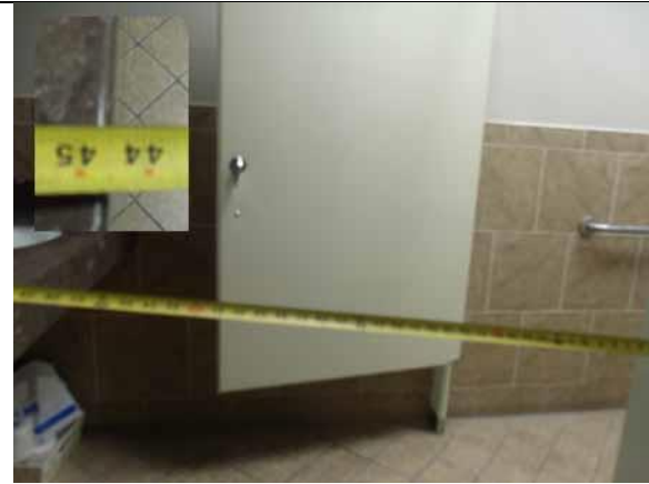
This access width is compliant
