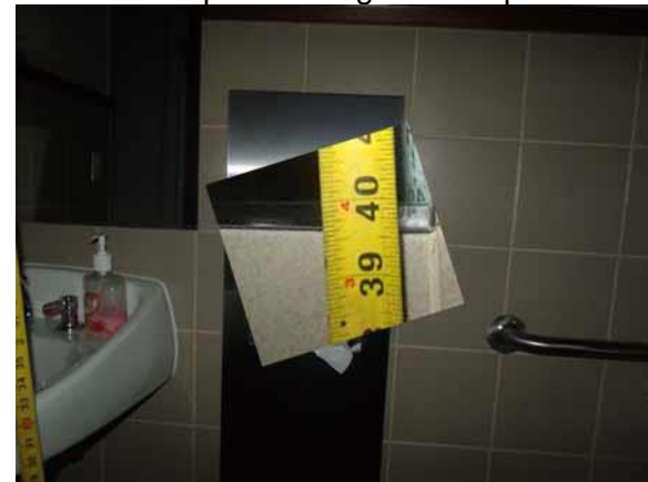
This dispenser height is compliant
