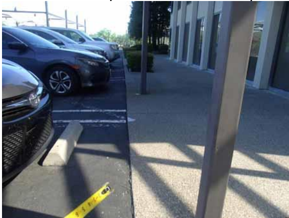
Provide a barrier between the accessible route and parking
