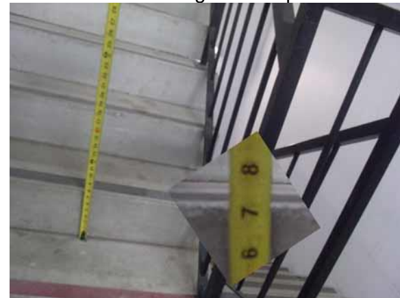
This riser height is compliant
