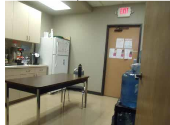
Provide proper exit braille signs typical of all exit route doors
