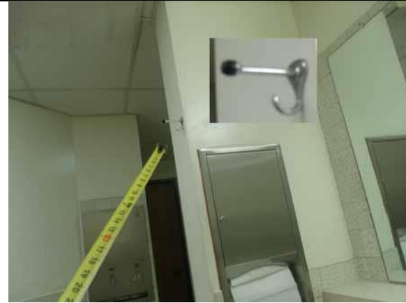
Provide a coat hook at 48" maximum high
