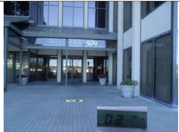
This section slope and width are compliant
