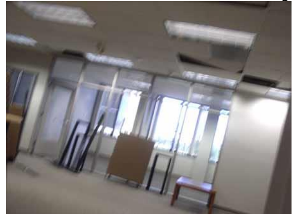
Maintain 44"-36" wide route when walls are installed
