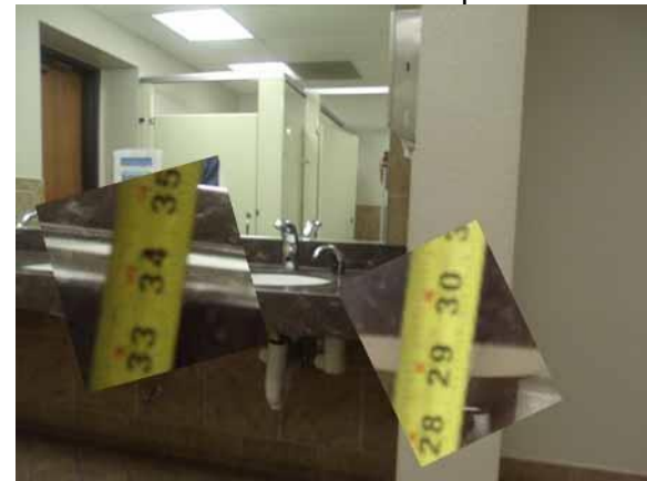
This lav height and knee clearance is compliant
