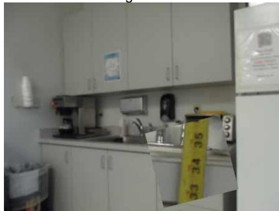
This counter height is compliant
