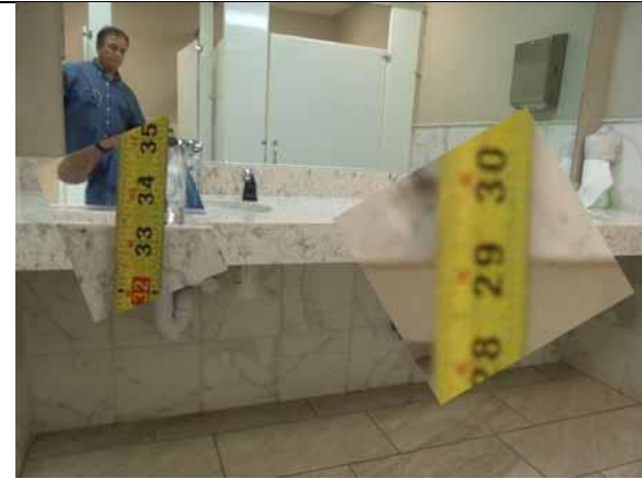
This lav height is compliant
