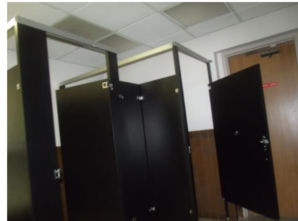
Overall two toilet stall shot
