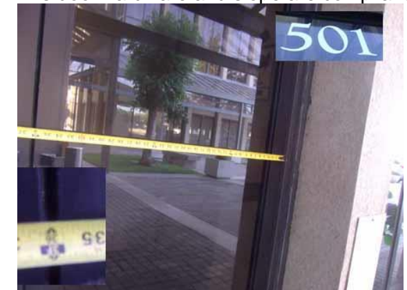
This door width is compliant
