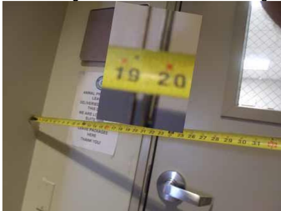
Maintain a minimum 18" strike side clearance
