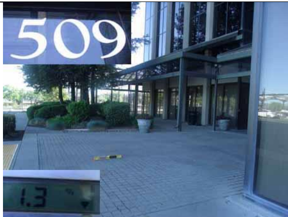
This section slope and width are compliant
