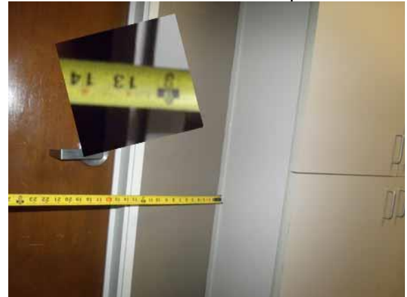
This push side clearance is compliant
