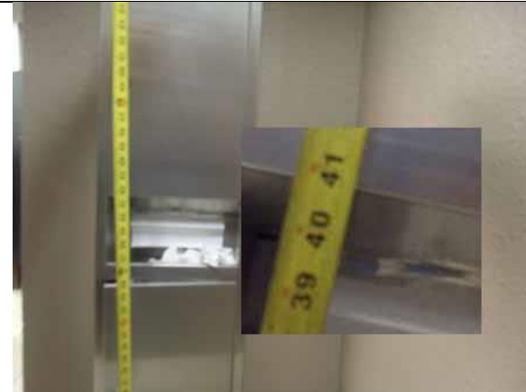
Maintain dispenser heights to be 40" maximum to operable parts
