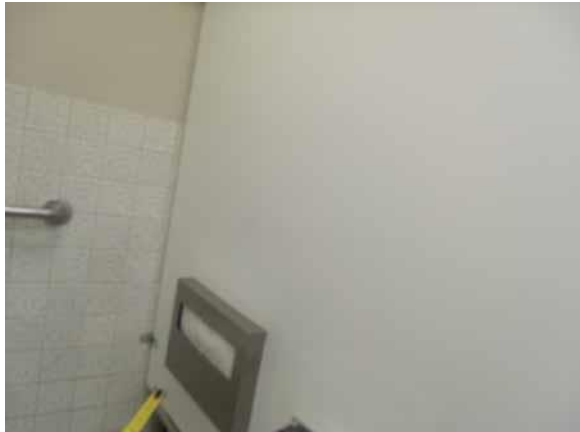
Properly locate the toilet seat cover dispenser
