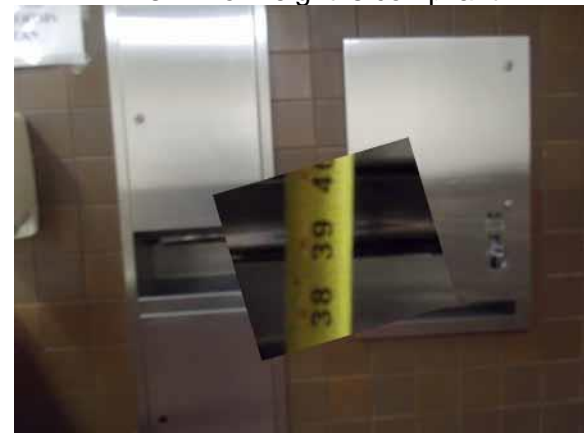
This paper towel dispenser location is compliant
