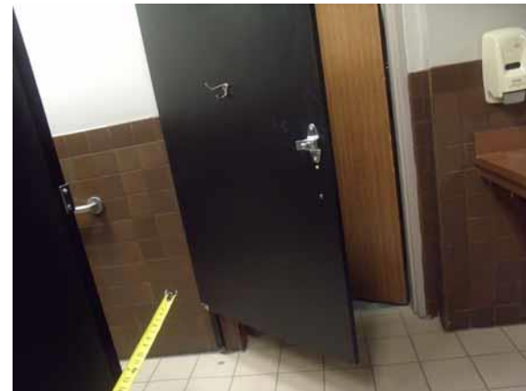
Stall doors shall be self-closing
