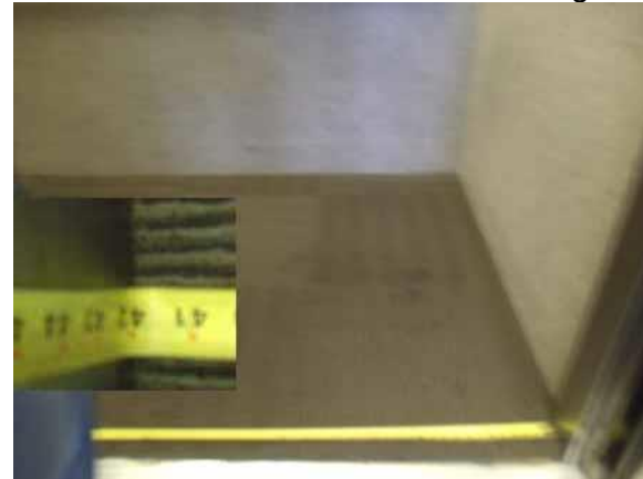
This opening width is compliant
