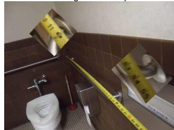
This side grab bar location is compliant
