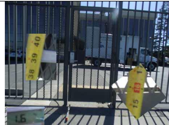
This door hardware and slope are compliant
