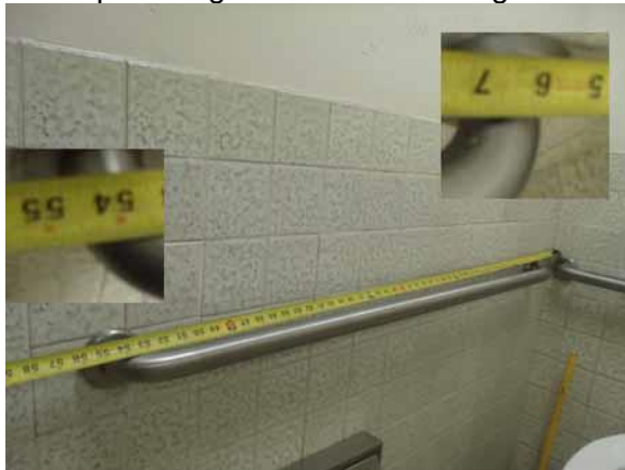
This side grab bar location is compliant
