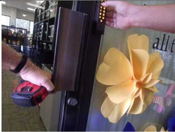
This type door handle is compliant
