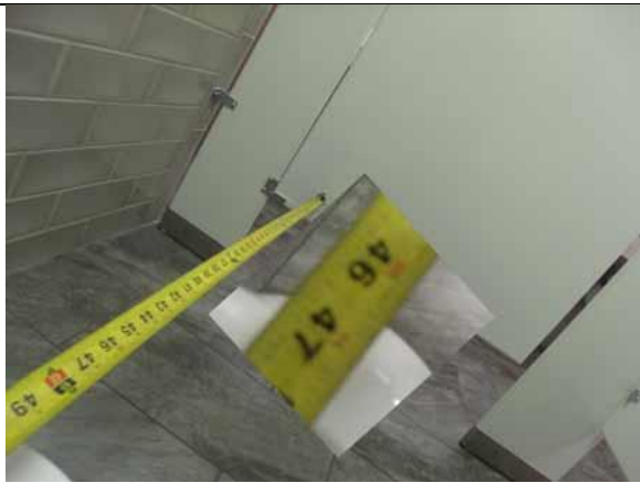
This distance shall be 48" minimum
