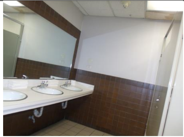
Overall Lav area
