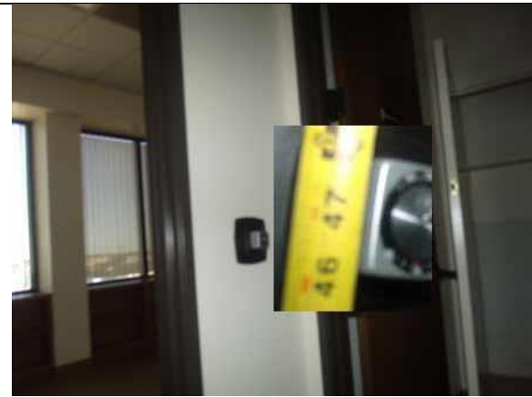
This control height is compliant
