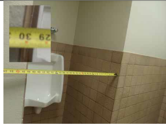
This width shall be 36" minimum
