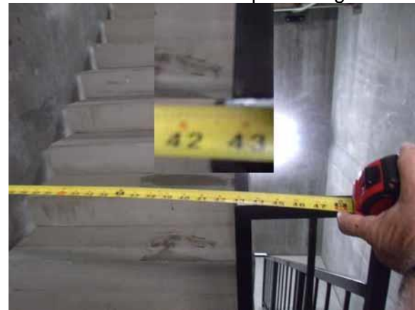
Stair width meets time of construction
