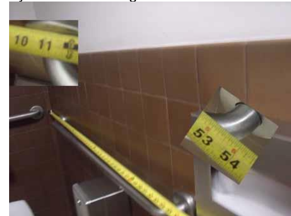
This side grab bar location is compliant
