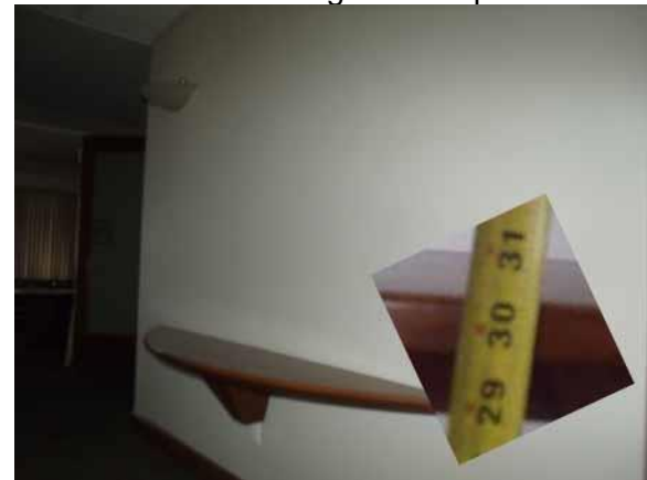
This counter height is compliant
