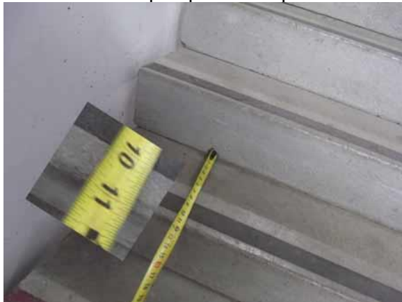
This step depth is compliant
