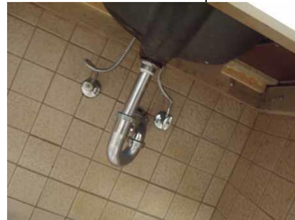
Properly protect the plumbing under the lav
