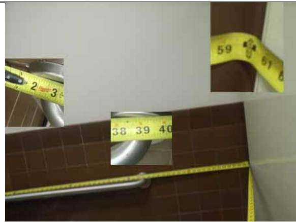
Properly locate the grab bars
