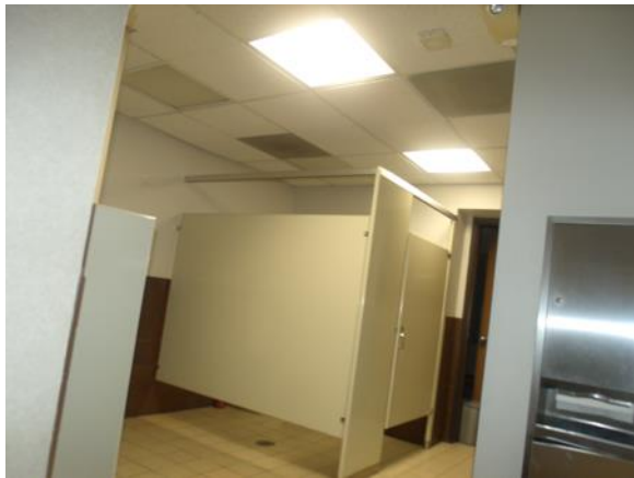
Overall stall area
