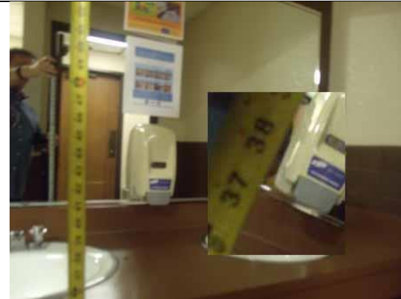
This dispenser height is compliant
