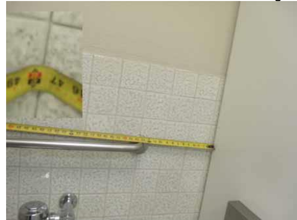
This stall width shall be 60" wide minimum
