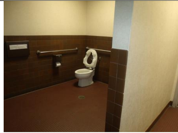
Over all toilet area
