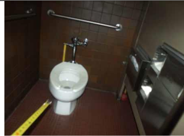
Provide proper toilet seat height
