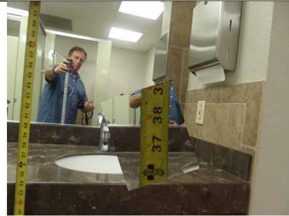
This mirror height is compliant
