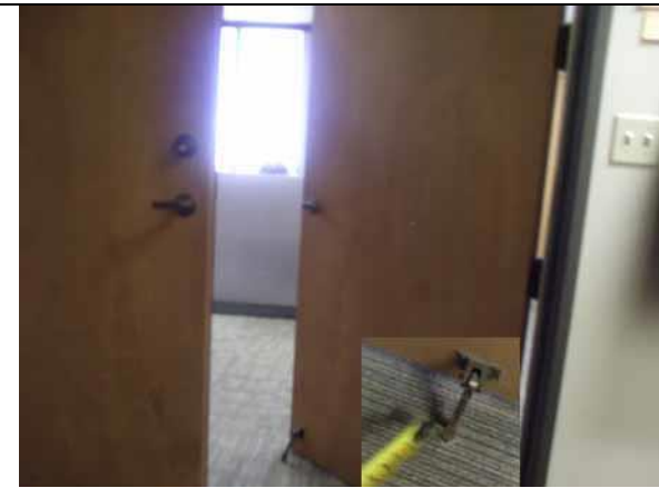
Remove the door stops from the bottom of the doors
