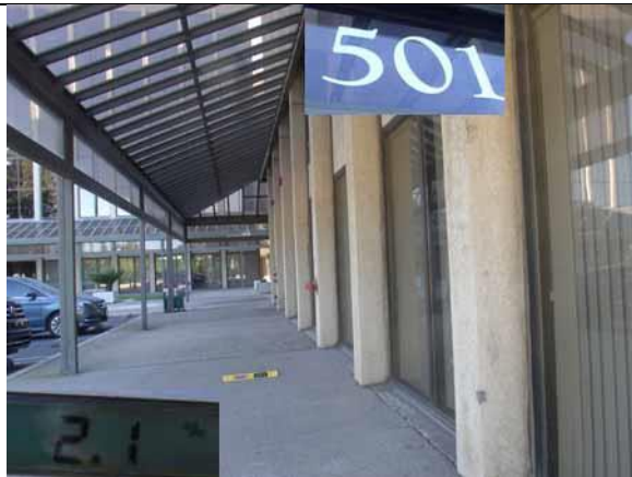
This section slope and width are compliant
