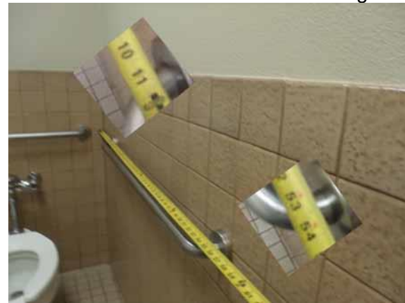
This side grab bar location is compliant
