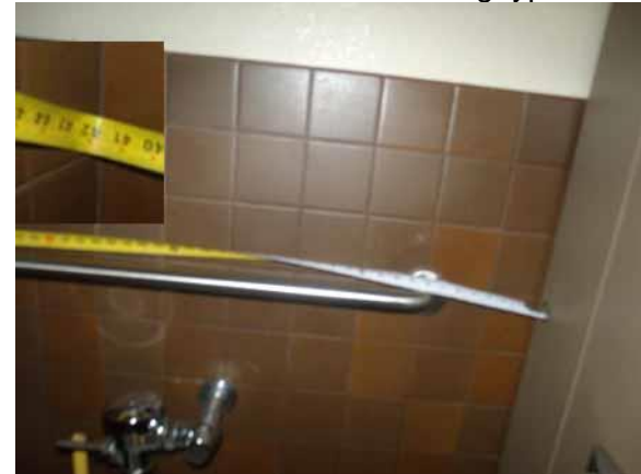
Toilet stall width shall be 60" wide minimum
