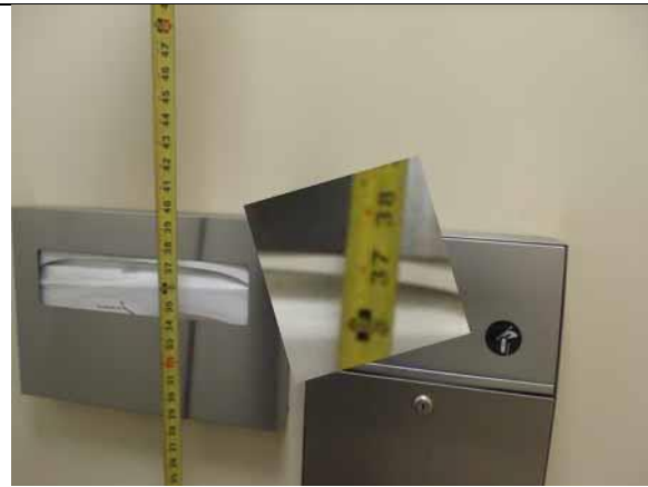
Toilet seat cover dispenser height is compliant
