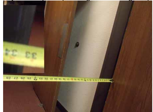
This door width is compliant
