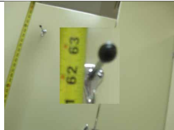
Provide a coat hook at 48" maximum high
