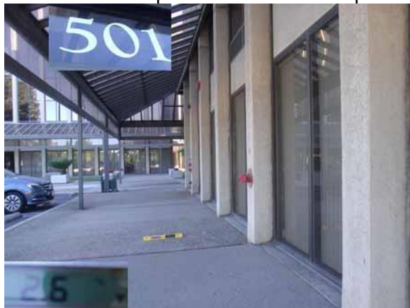
This section of cross slope exceeds 2.08%
