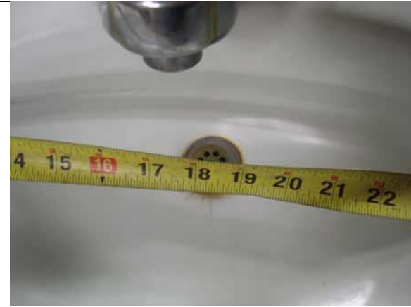
This lav offset is compliant
