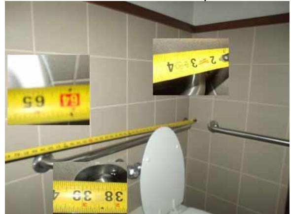
Properly locate the rear grab bar
