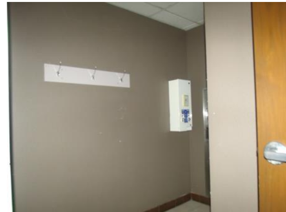
Overall entrance shot
