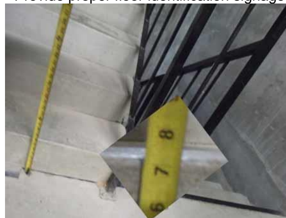
This riser height is compliant with applicable code
