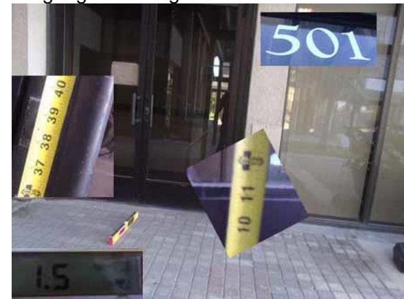
This door hardware and slope are compliant
