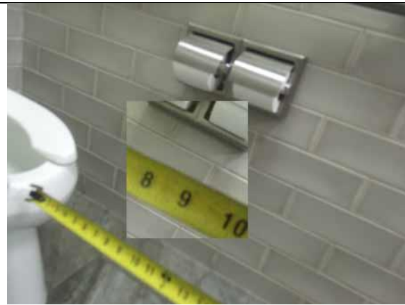
This toilet paper location is compliant
