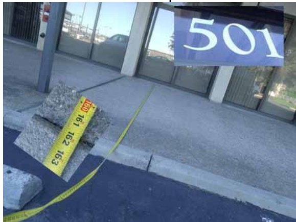
This is the width of the route to be repaired
