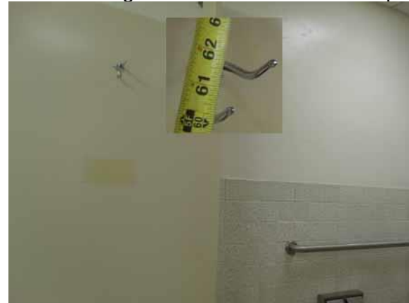
Provide a coat hook at 48" maximum high
