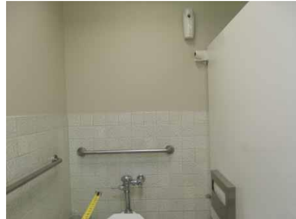
Properly locate the rear grab bar
