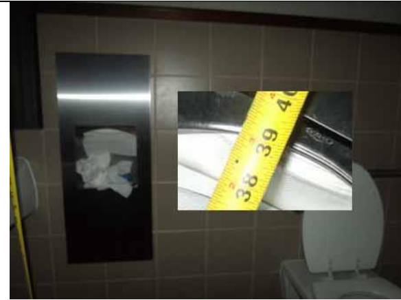
This dispenser height is compliant
