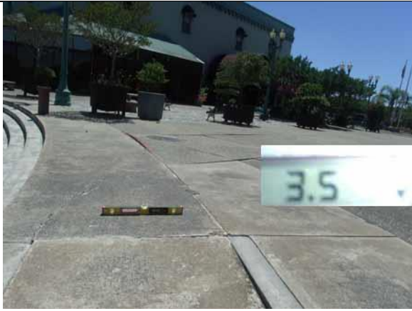
This top landing exceeds 2.08% cross slope
