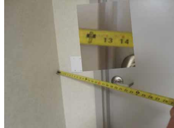
This push side clear area is compliant
