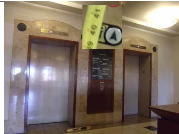
This call button height is compliant
