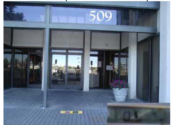
This section slope and width are compliant
