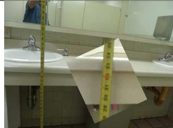
This lav height is compliant
