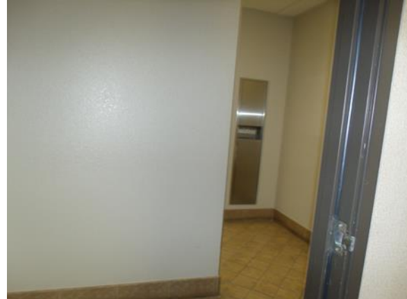
Overall entrance shot
