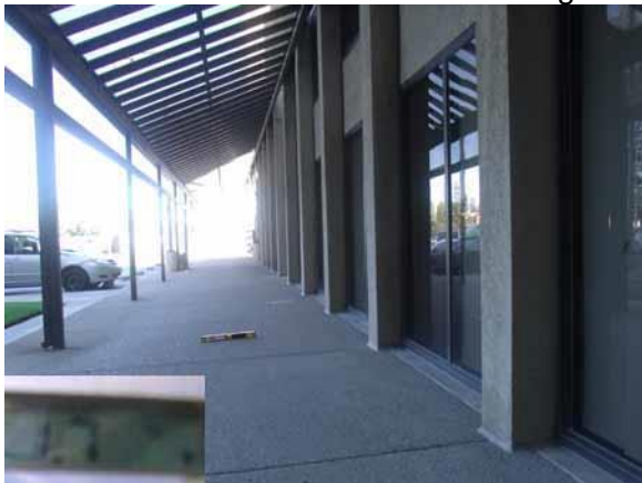
This section slope and width are compliant
