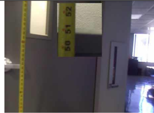
Lower viewing window in doors to 43" high maximum typical
