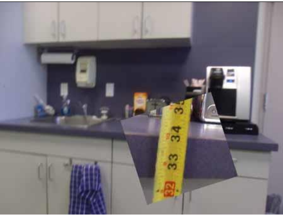
This counter height is compliant
