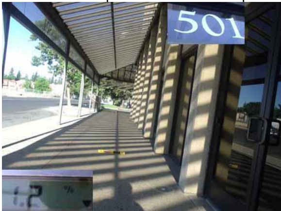
This section slope and width are compliant
