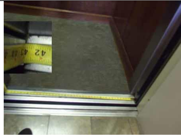
This opening width is compliant
