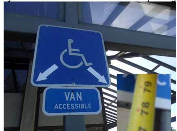
This signage is not compliant
