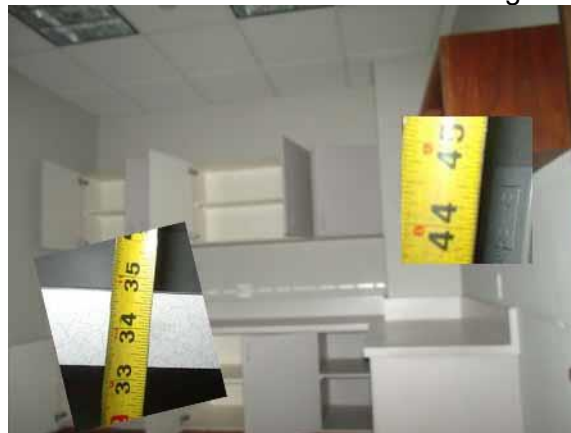
Extend electrical at counters to be within reach ranges
