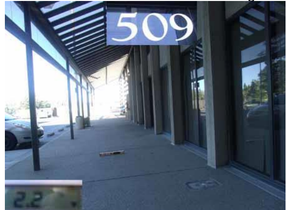
This section slope and width are compliant
