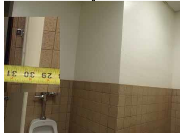
This width shall be 30" wide minimum
