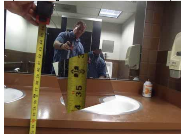
Maintain mirror height to be 40" maximum to reflective parts
