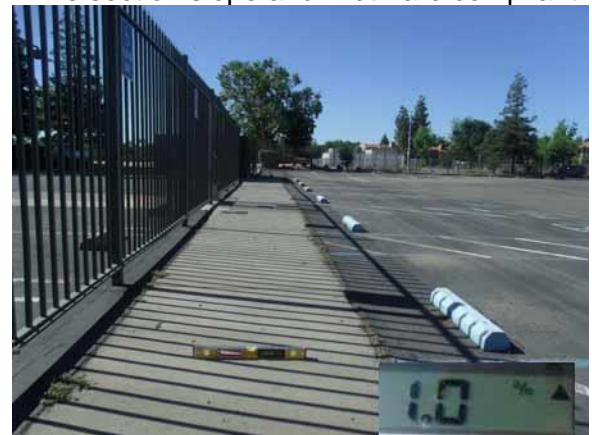
This section slope and width are compliant
