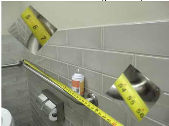
This side grab bar location is compliant
