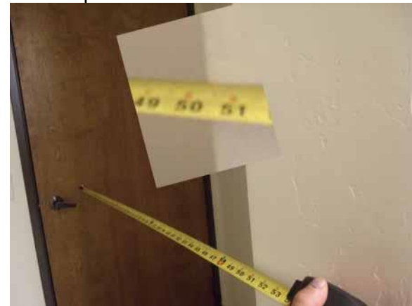
Reverse the door to swing out of the restroom area
