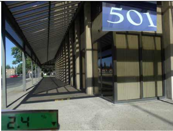
This section of cross slope exceeds 2.08%
