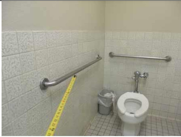
Properly locate the grab bars
