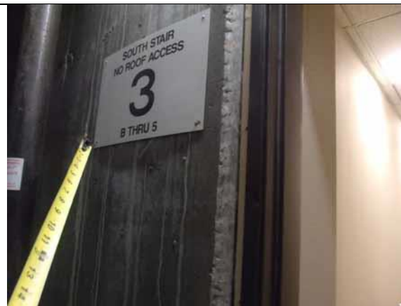
Provide proper floor identification signage
