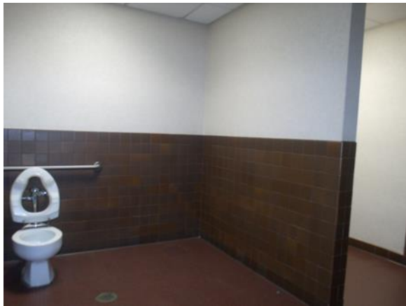
Over all toilet area
