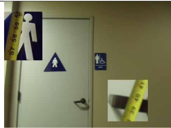
These heights are compliant
