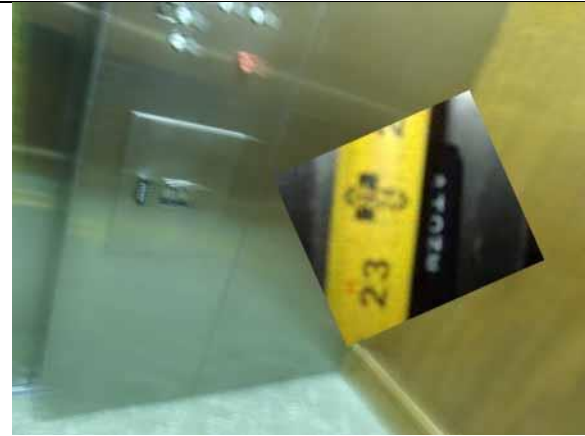
This height is compliant
