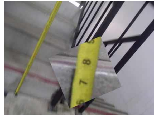
This riser height is compliant
