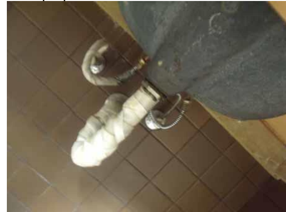
Maintain plumbing protection under lavs
