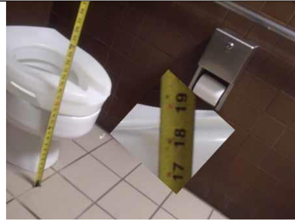
This toilet seat height is compliant
