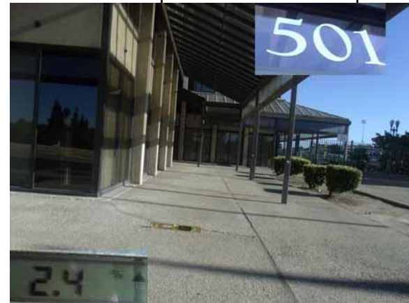
Provide sign directing to the accessible route/entrance
