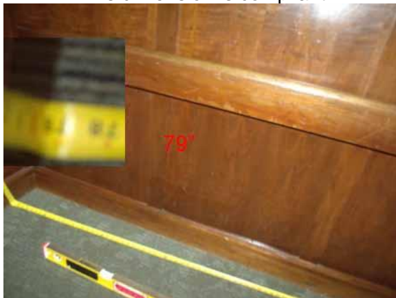
This dimension is compliant without base molding
