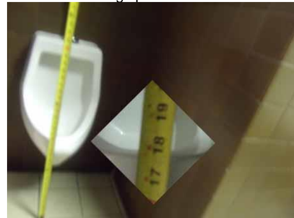
This urinal exceeds 17" high to top of rim
