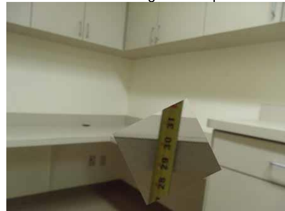
This counter height is compliant
