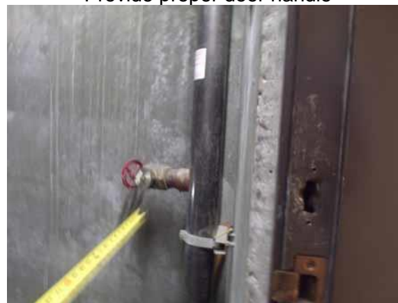
Provide cane detection under hose connection
