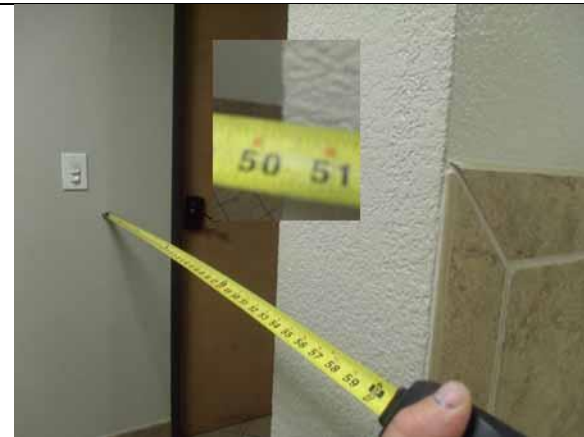
This clear width is compliant
