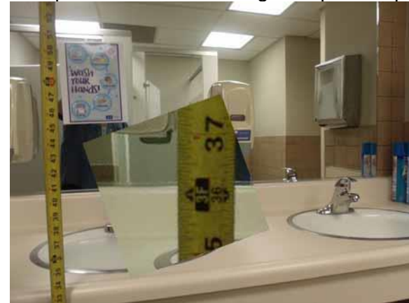
This mirror height is compliant
