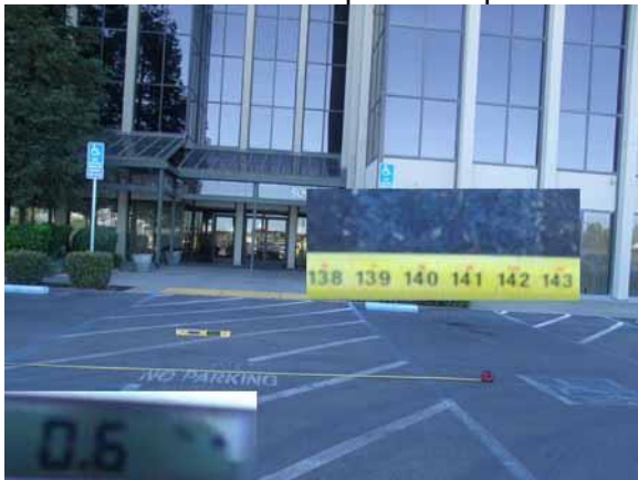
This accessible access aisle width and slope are compliant
