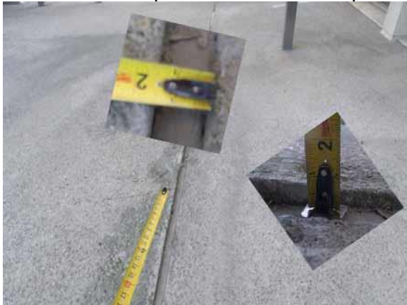
Repair the damaged wood gap
