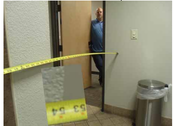
This clear width is compliant
