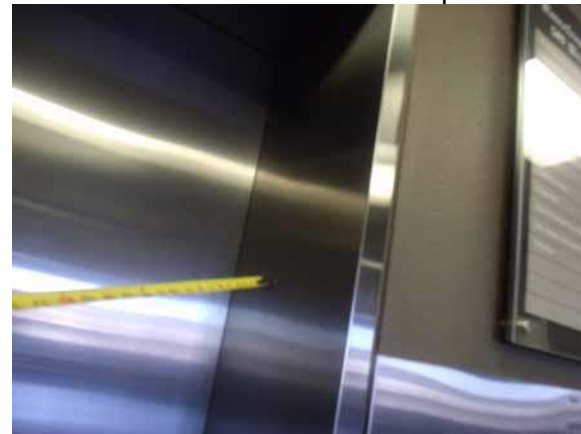
There is no 2" star for ground floor on the elevator door jambs
