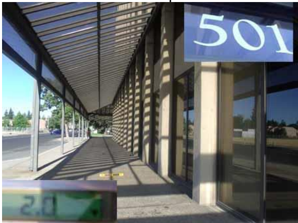
This section slope and width are compliant
