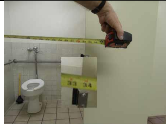
This door width is compliant
