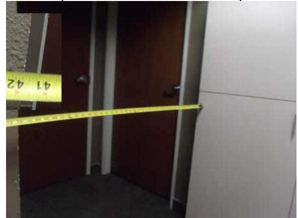
Remove cabinet for proper 44" wide access
