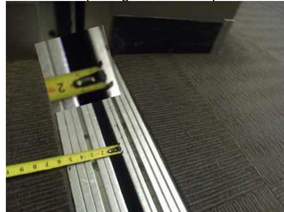
This gap is compliant
