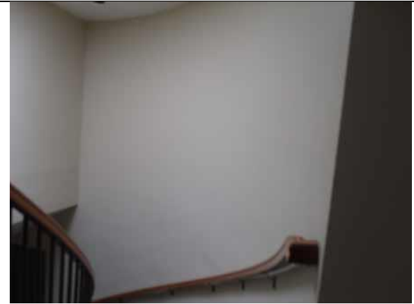
Interior stairs between 4 th and 5 th floors
