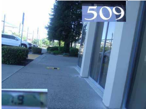
This section slope and width are compliant
