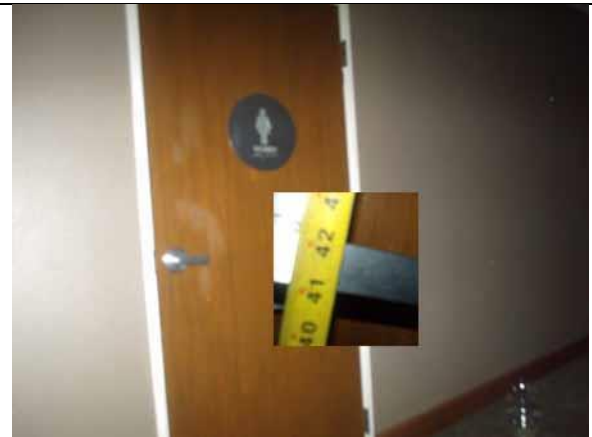
This door handle is compliant
