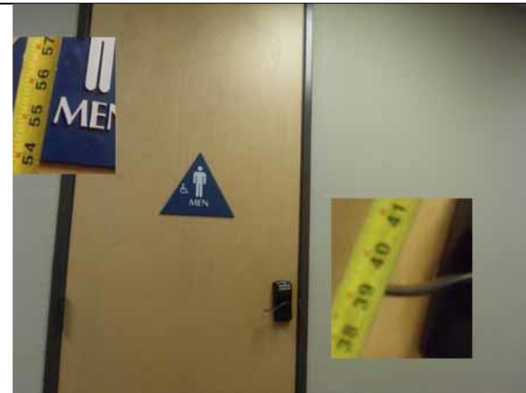
These heights are compliant
