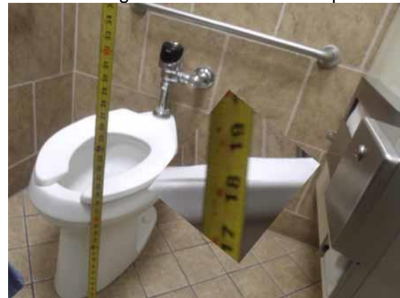
This toilet seat height is compliant
