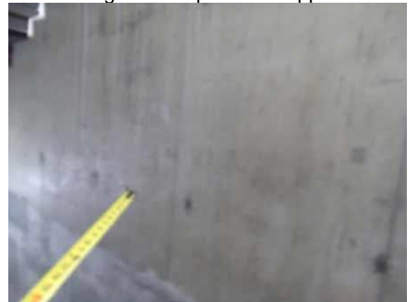
Handrails are not provided on both sides
