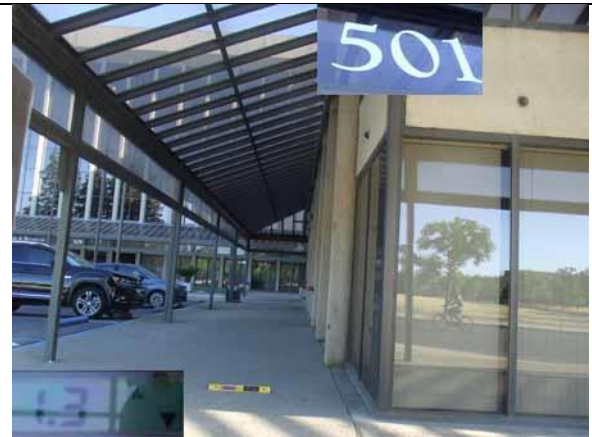
This section slope and width are compliant
