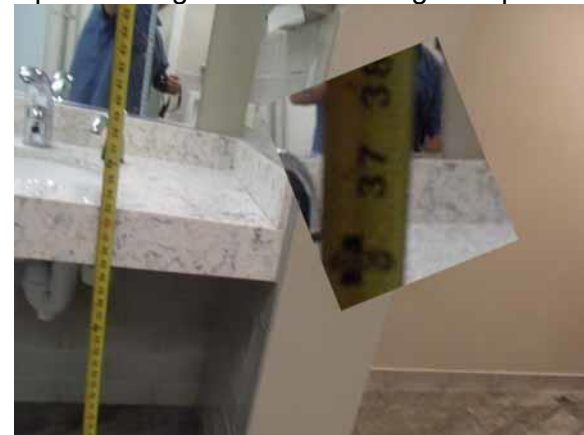
This mirror height is compliant
