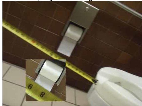
This toilet paper location is compliant
