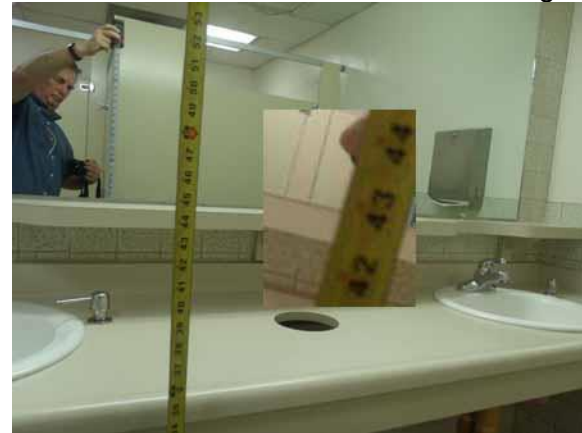
This mirror height exceeds 40" to reflective parts
