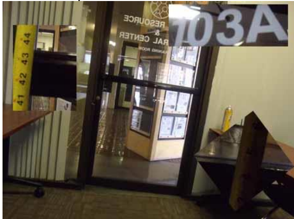
A minimum 10" high smooth solid kick plate required on doors
