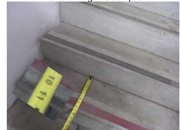
This step depth is compliant
