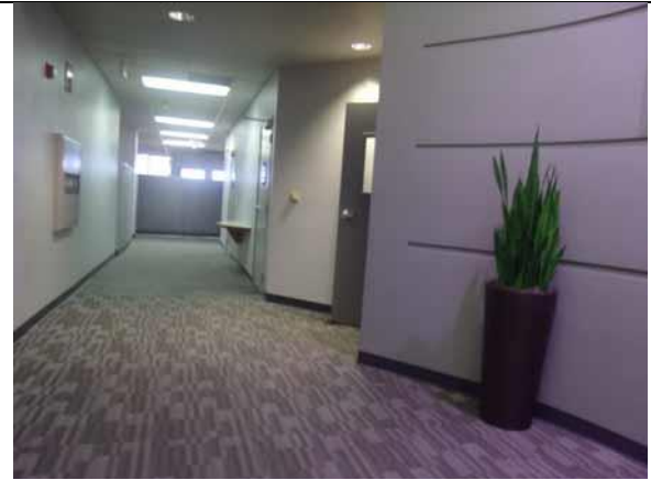
Maintain a min 44" wide route or 32" min for 24" long max in corridors
