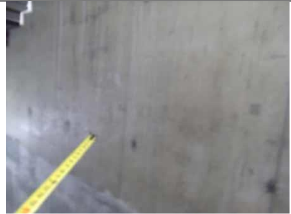
Handrails are not provided on both sides
