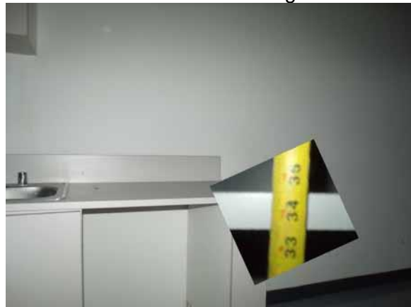
This counter height exceeds 34" high if alteration is performed
