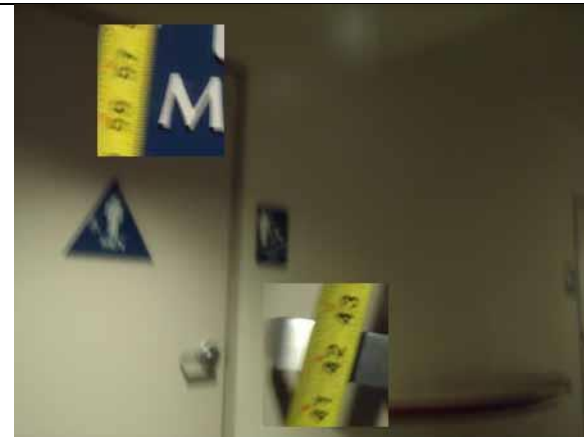
This door hardware is compliant
