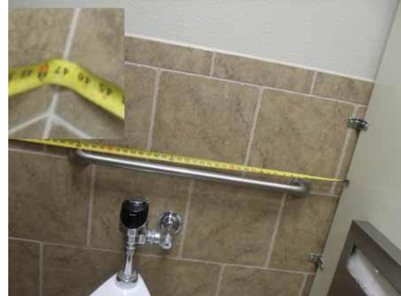
Toilet stall width shall be 60" wide minimum
