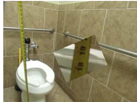
This toilet seat height is compliant
