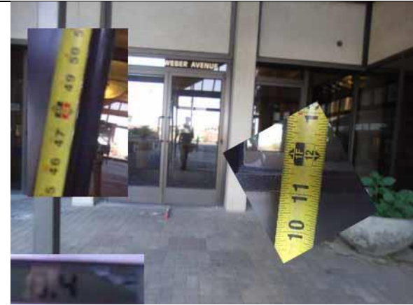
This door hardware and slope are compliant
