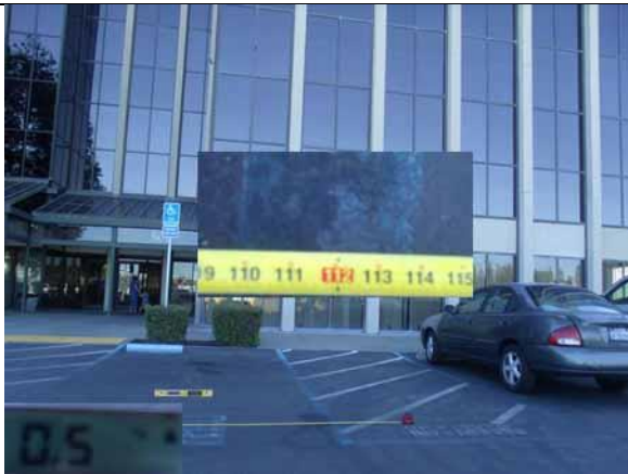
This accessible parking width and cross slope are compliant
