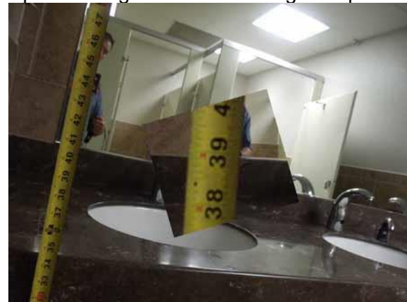
This mirror height is compliant
