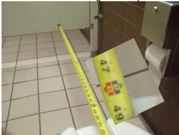
This distance in front of the toilet is compliant
