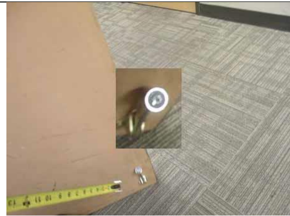
Remove door stops from the bottom of all doors
