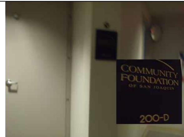
Provide proper room identification braille signage Typical
