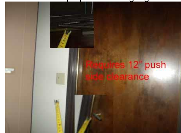
Move door down for proper side clearances
