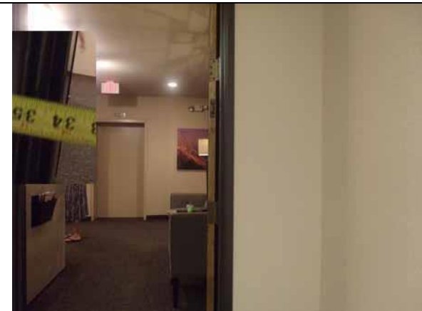
This clear opening width is compliant
