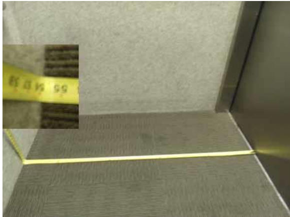
This dimension is compliant
