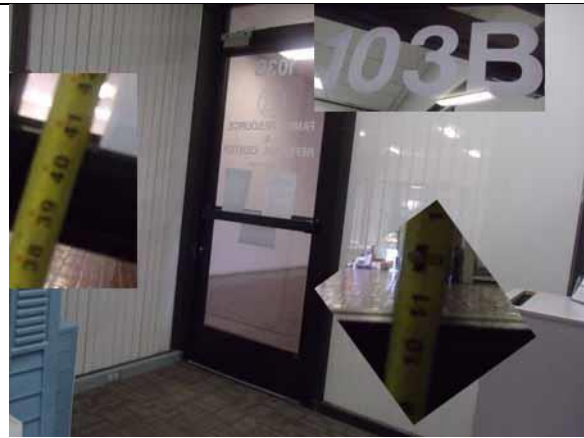
This door hardware is compliant
