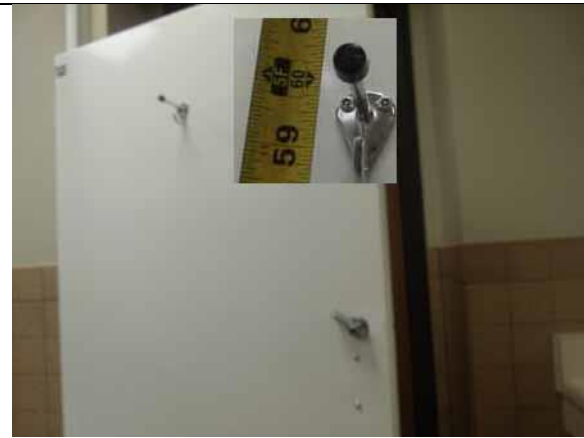
Coat hook shall be 48" maximum high
