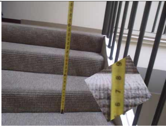
This riser height shall be 7" maximum
