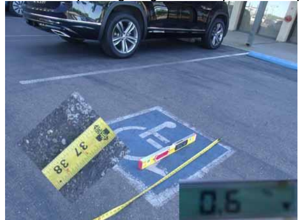
This symbol size does not meet MUTC requirements
