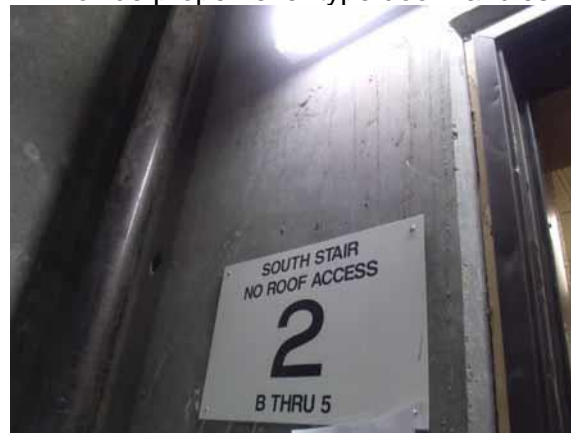
Provide proper floor identification sign
