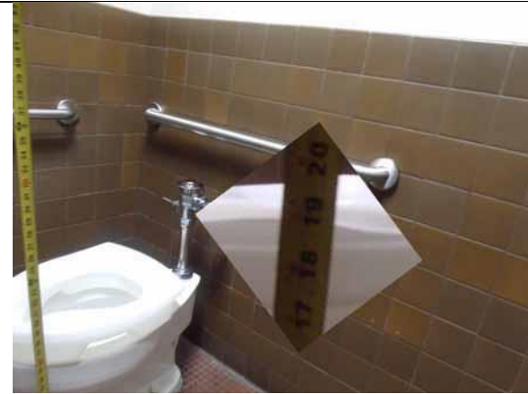
This toilet seat height is compliant
