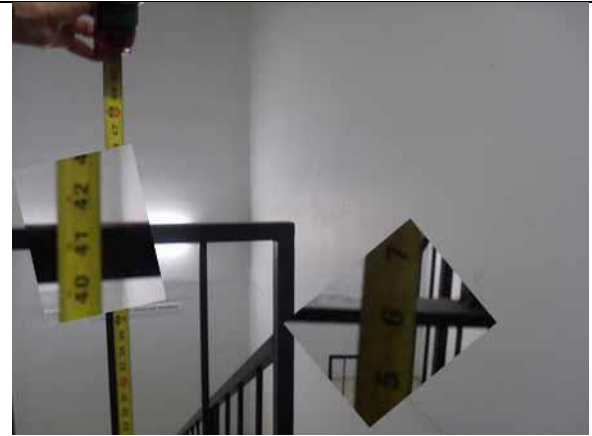
This guard height is not 42" minimum
