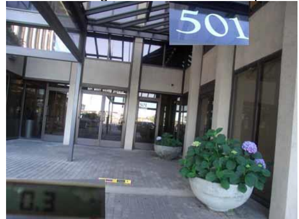
This section slope and width are compliant
