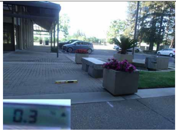
This section slope and width are compliant
