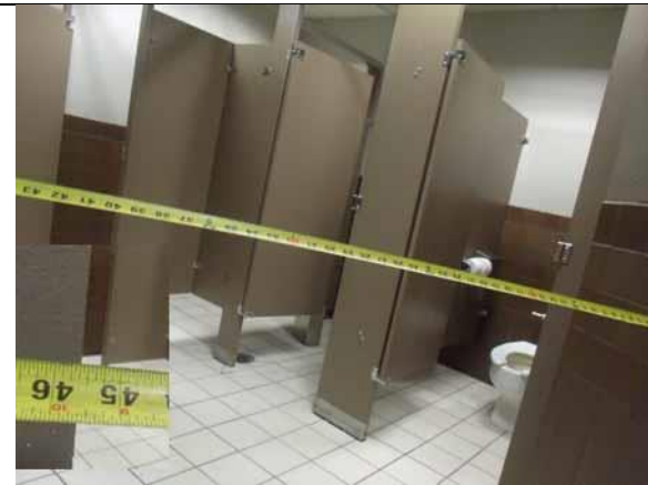
This width to the accessible stall is compliant
