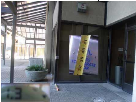
This push pad height is compliant
