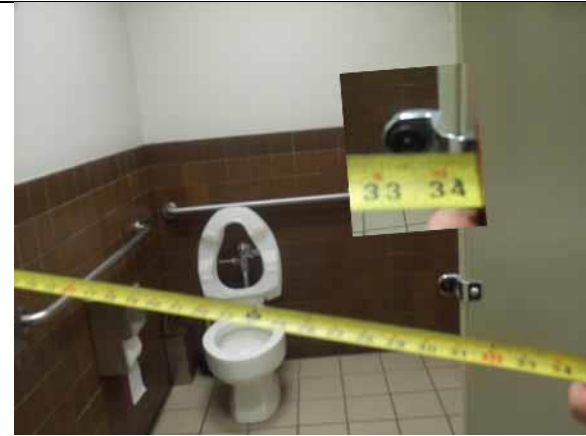
This clear opening width is compliant
