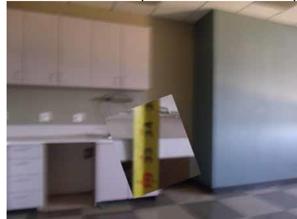
This counter height is compliant
