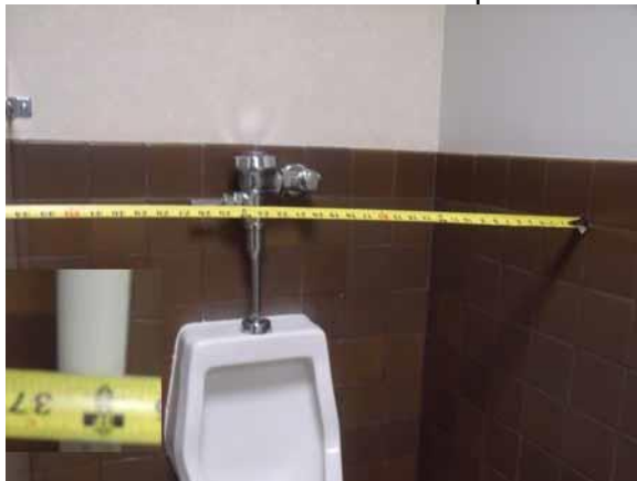
This width shall be 36" wide minimum
