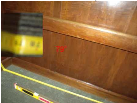
This dimension is compliant without base molding
