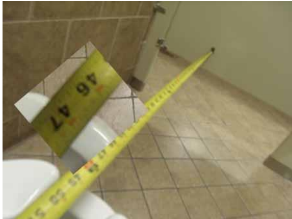
This clear length shall be 48" minimum
