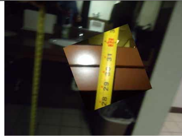
Provide proper knee clearance under the lav
