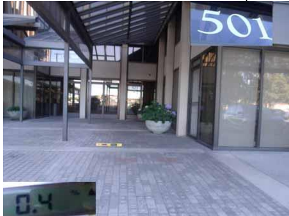
This section slope and width are compliant
