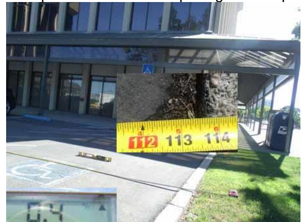
Properly mark and maintain the accessible parking areas
