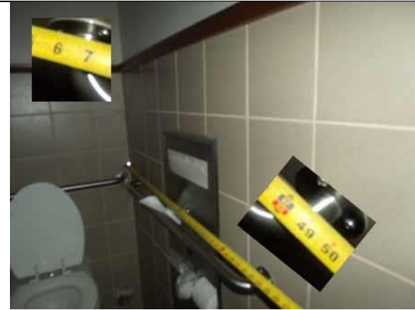
Properly locate the side grab bar
