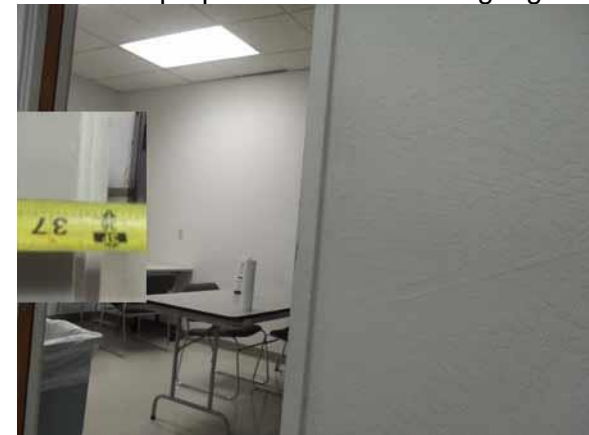
This clear opening width is compliant
