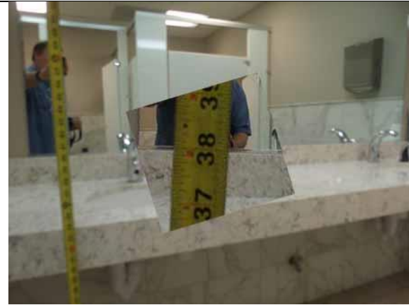
This mirror height is compliant
