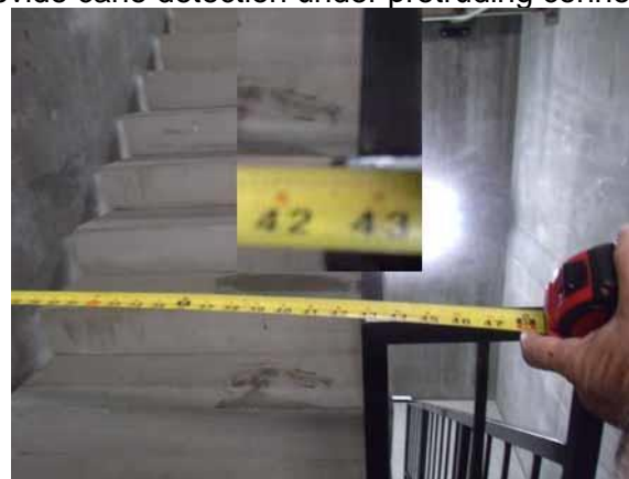
Stair width meets time of construction
