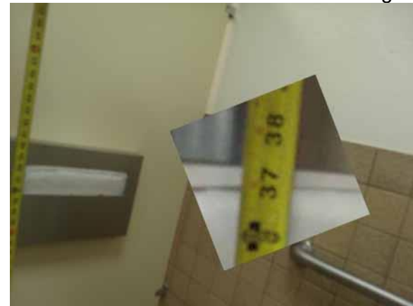
This dispenser height is compliant
