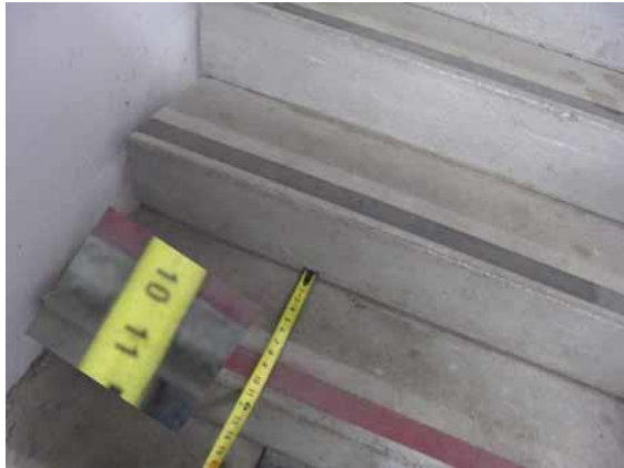
This step depth is compliant
