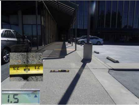
This section slope and width are compliant
