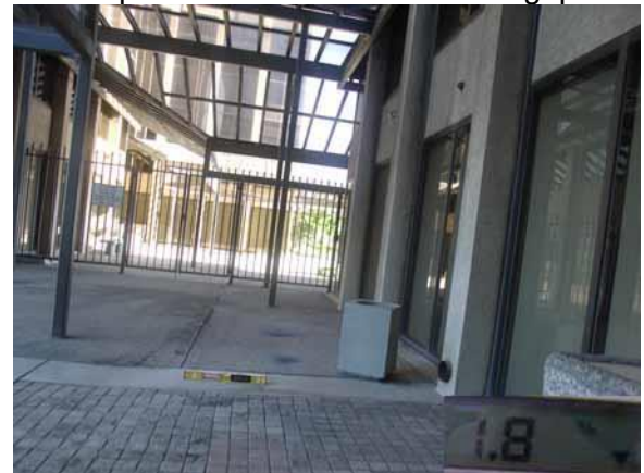
This section slope and width are compliant
