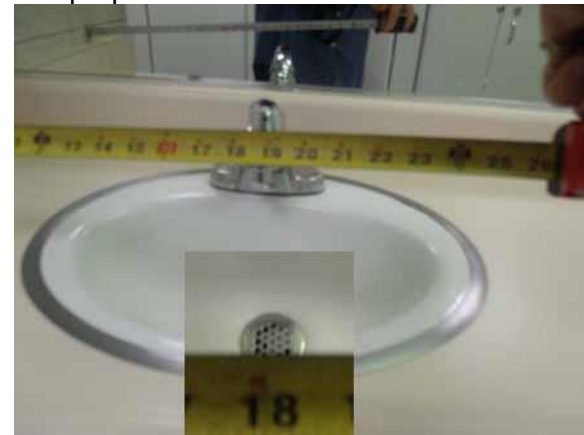
This lav offset is compliant
