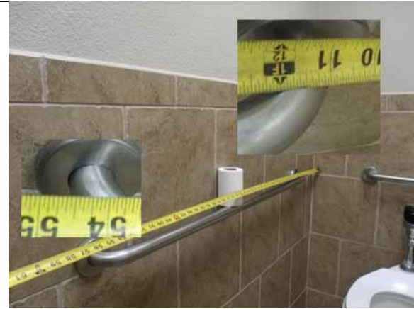
This side grab bar location is compliant
