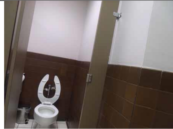
Remove stall panel and make a 60" wide stall
