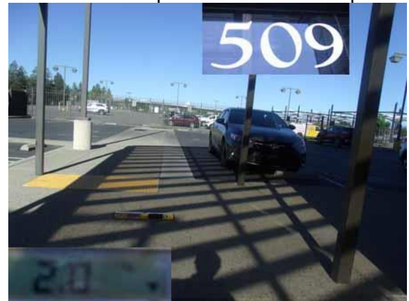
This section slope and width are compliant
