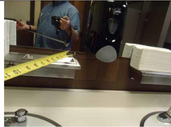
The soap dispenser exceeds 40" high to operable parts
