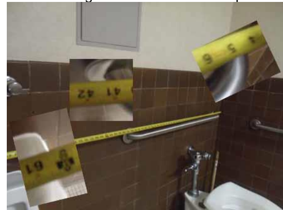
Properly locate the rear grab bar
