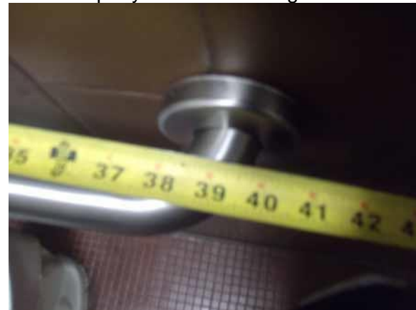
Properly locate the rear grab bar
