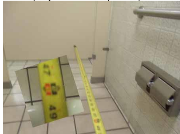
This length is compliant
