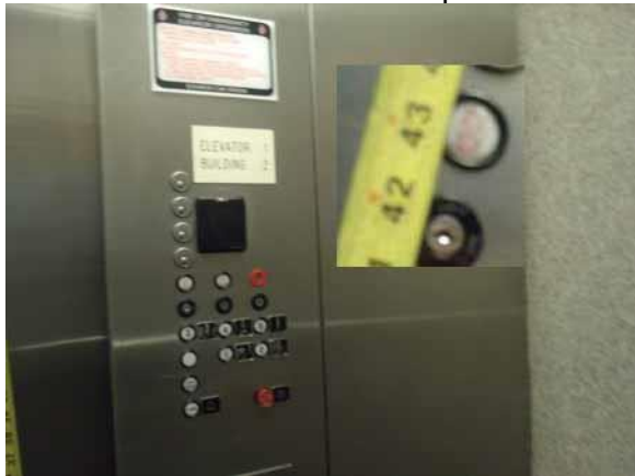
This control height is compliant
