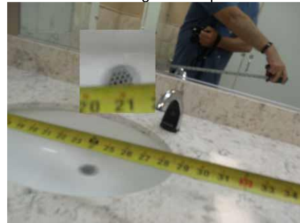
This lav offset is compliant
