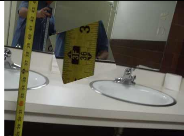
This mirror height is compliant
