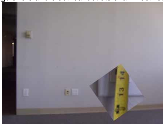
This outlet meets federal requirements for 1991 standards
