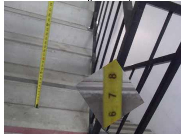
This riser height is compliant
