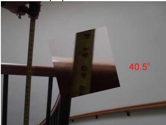
This guard height is not 42" high minimum
