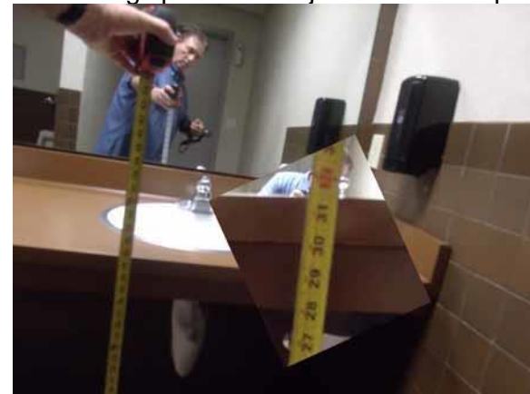
Provide proper knee clearance under the lav
